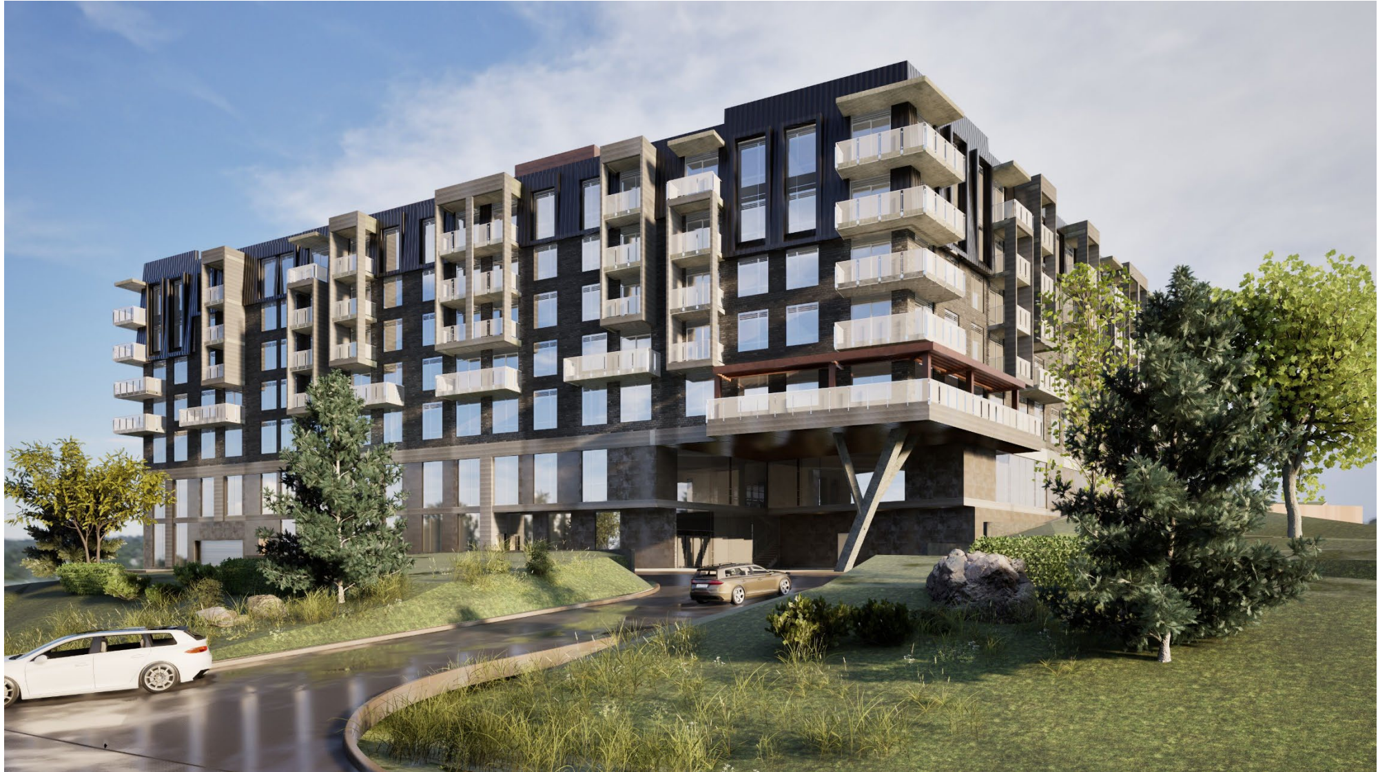
View Looking West from Highway 27
