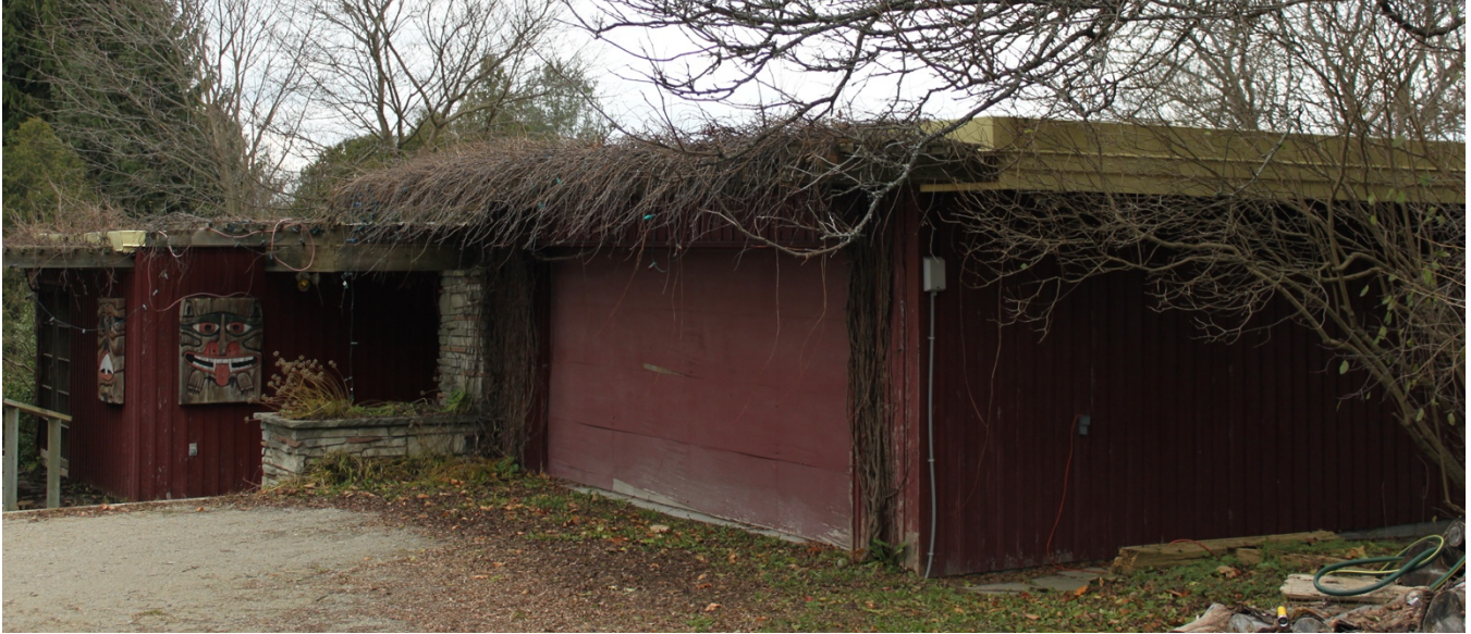
view of garage (2012)
