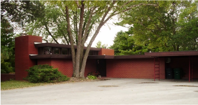
Trier House, built 1967
