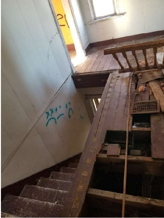
Pic. 21, Pic. 22: Broken Floor, Ceiling, and Stair Guard Rails
