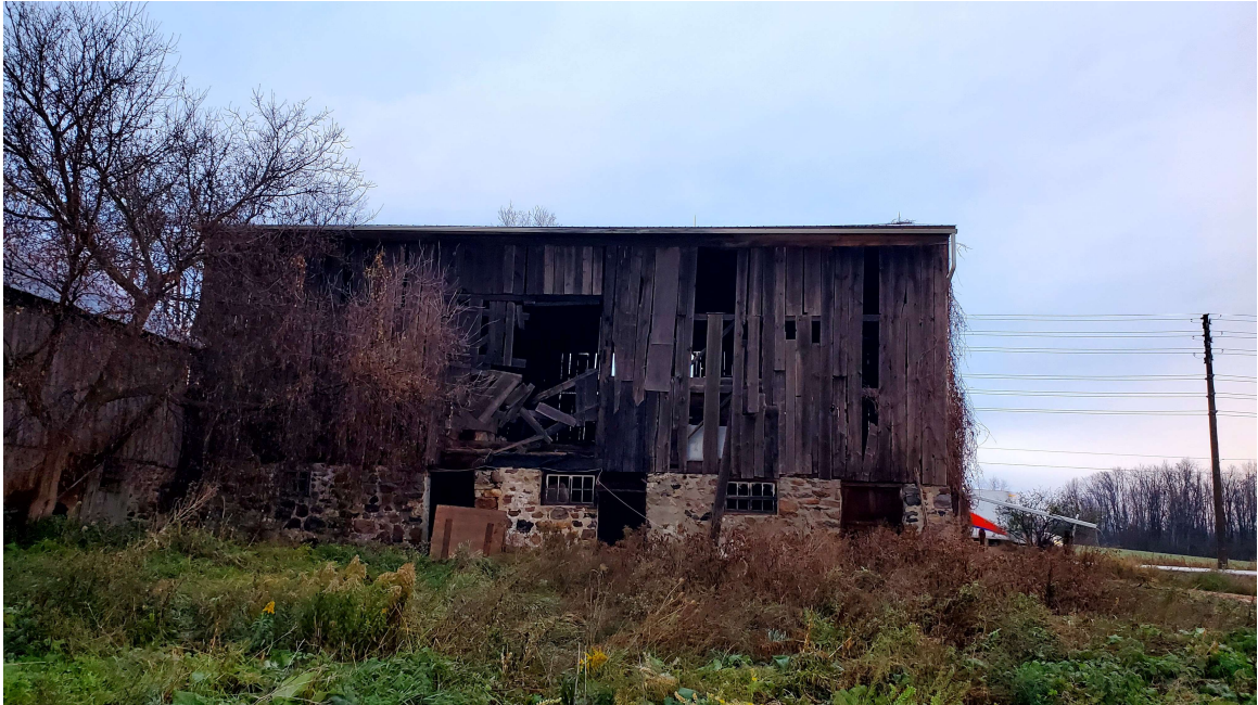
Pic. 26: Backside of the Barn
