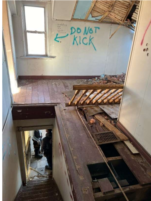
Pic. 21, Pic. 22: Broken Floor, Ceiling, and Stair Guard Rails
