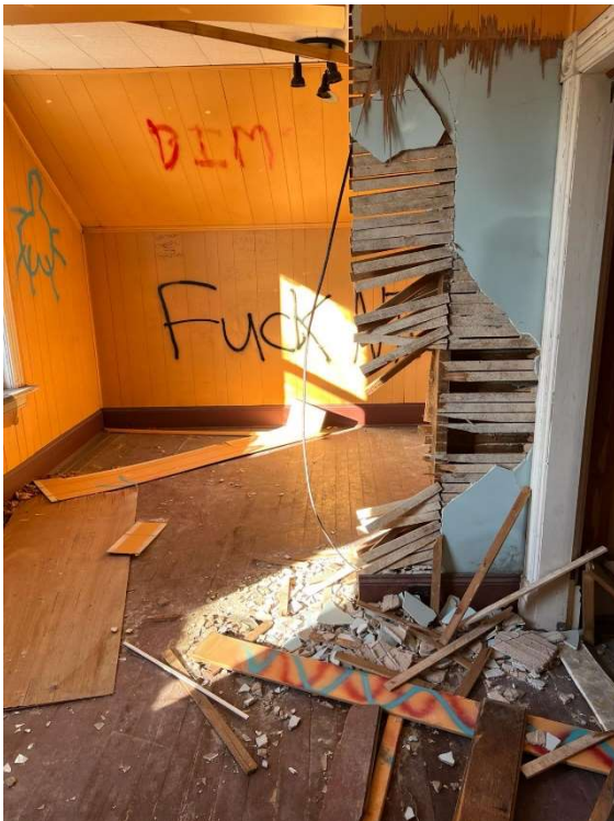
Pic. 17, Pic. 18: Broken and Deteriorated Ceiling, Damp and Decay wood floor and Debris
