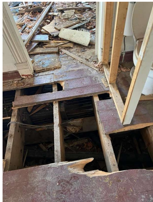
Pic. 23, Pic. 24: Broken Floor and Stair Guard Rails with Debris
