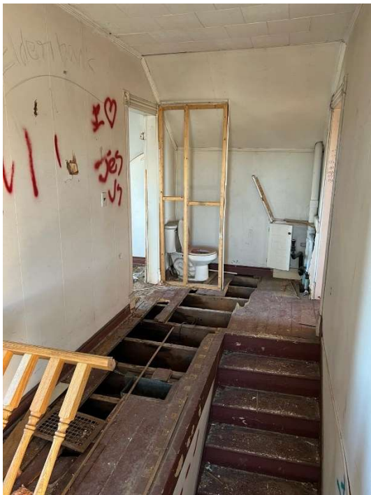
Pic. 23, Pic. 24: Broken Floor and Stair Guard Rails with Debris
