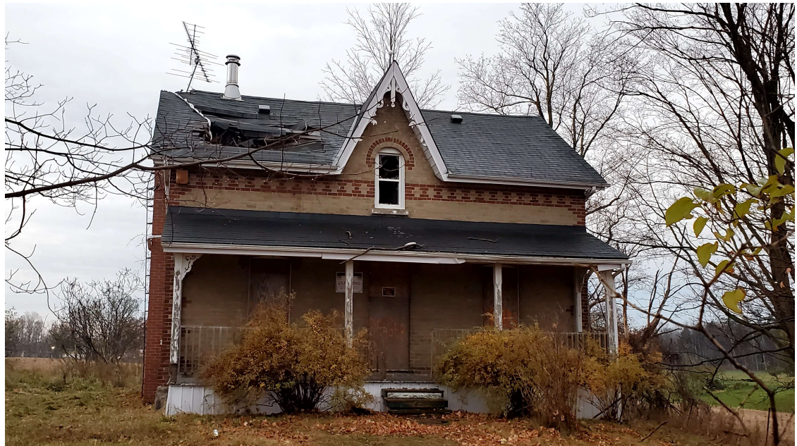
Pic. 2: Heritage House-Northwest
