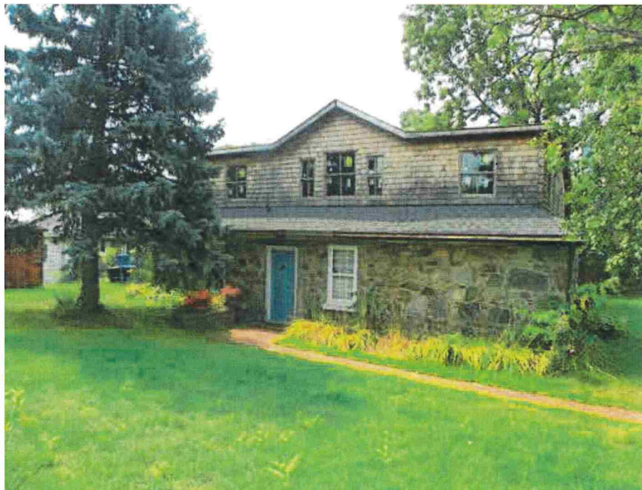
Figure 18: The east façade of Joshua Oliver House.
