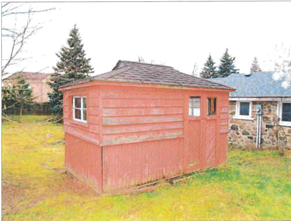
Figure 30: View facing southwest of Outbuilding 2.
