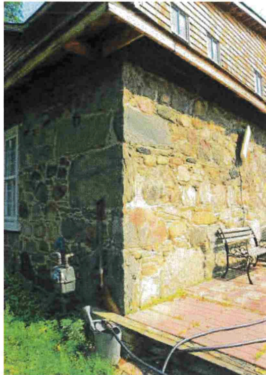
Figure 17: The southwest corner of Joshua Oliver House showing the large stone quoins and coursed rubble masonry.
