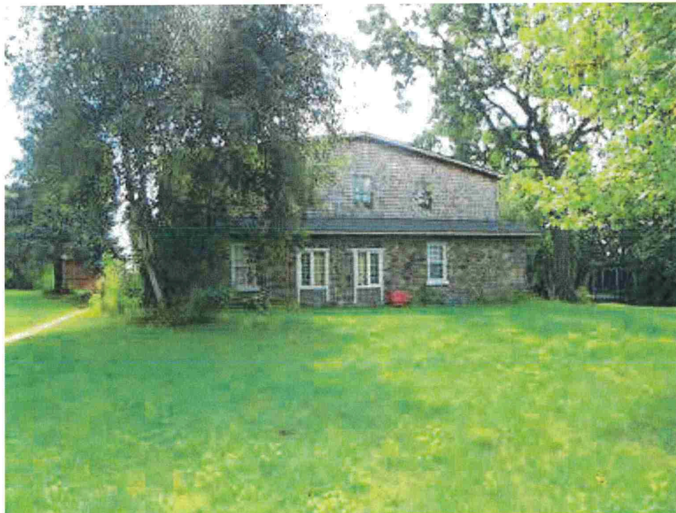
Figure 16: The north façade of Joshua Oliver House.
