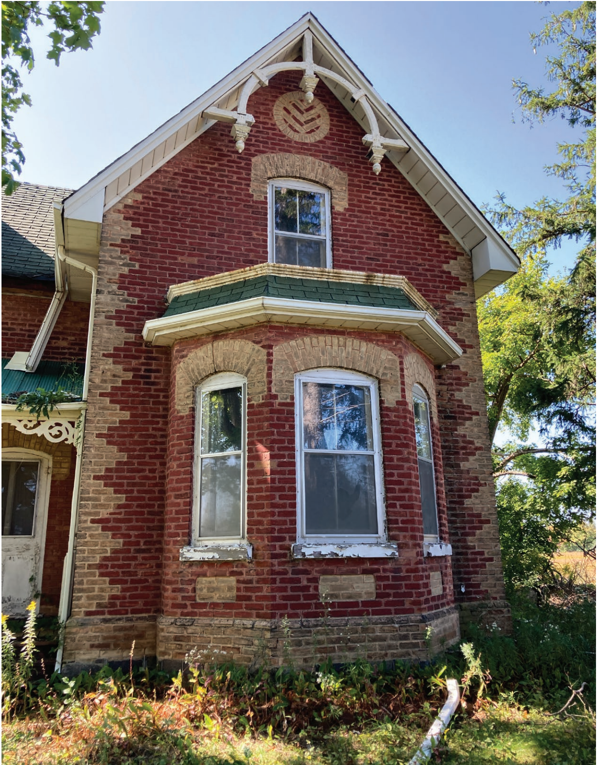
East elevation of the two-storey brick farmhouse (ERA, 2023).
