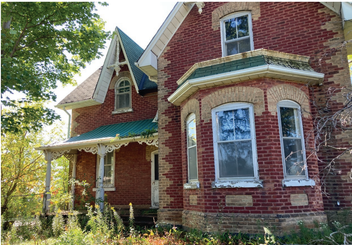
East elevation of the two-storey brick farmhouse (ERA, 2023).
