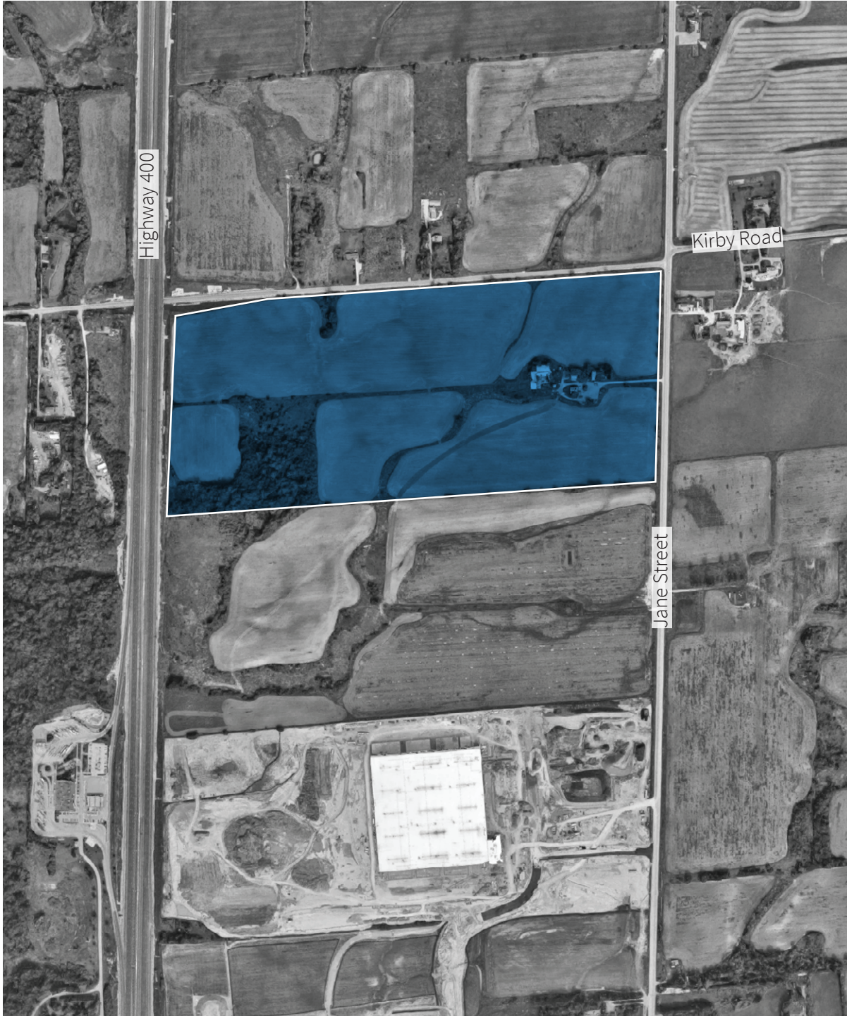
Aerial image showing the Site, shaded blue. Note that the barns/outbuildings captured in this image have since been demolished (Google, 2023; annotated by ERA).
