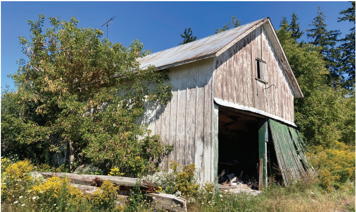
South and west elevation of the one-storey garage (ERA, 2023).
