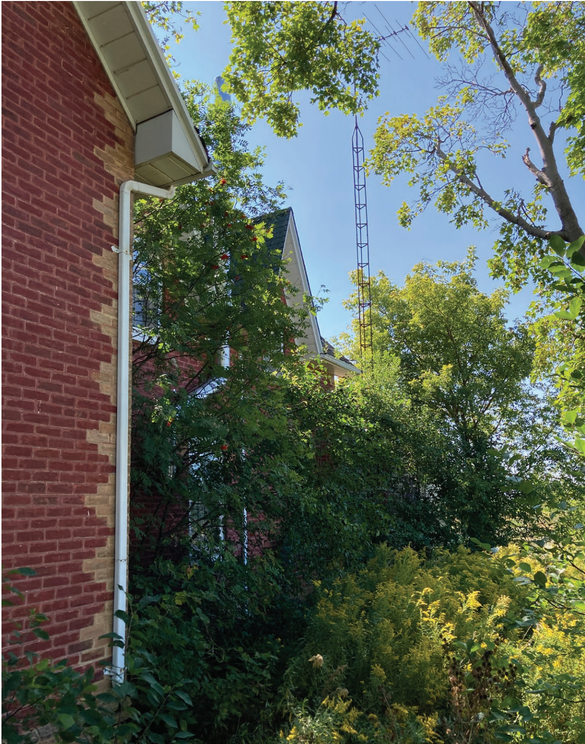
North elevation of the two-storey brick farmhouse (ERA, 2023).
