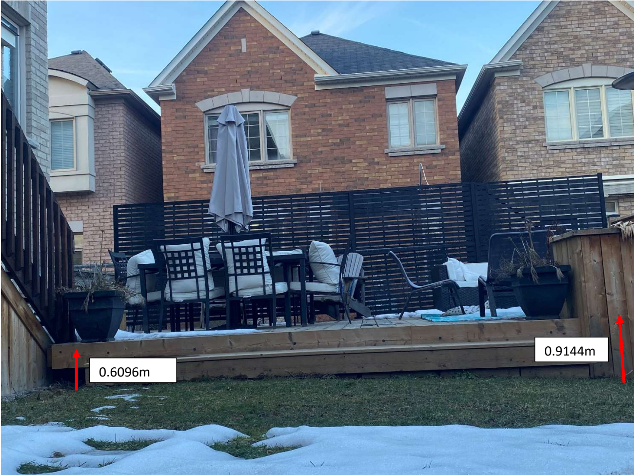
North facing view
