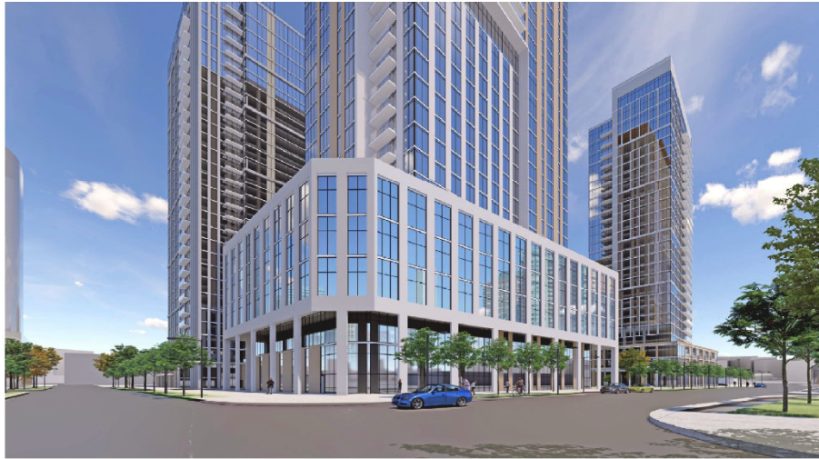
Look From North West at Intersection of White Elm Road and Maplecrete Road
