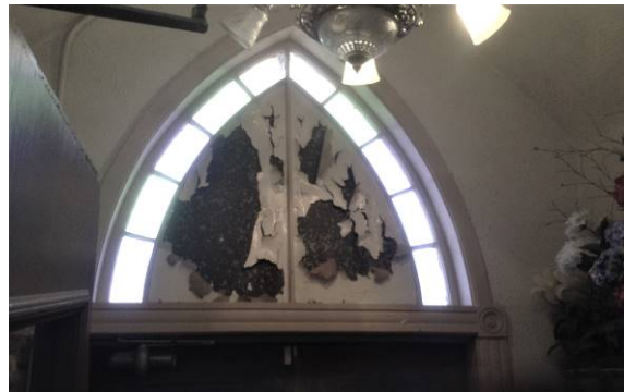
Figure 12. Interior of ogee transom window.
