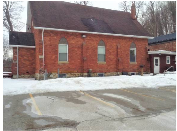
Figure 15. View from the north.
