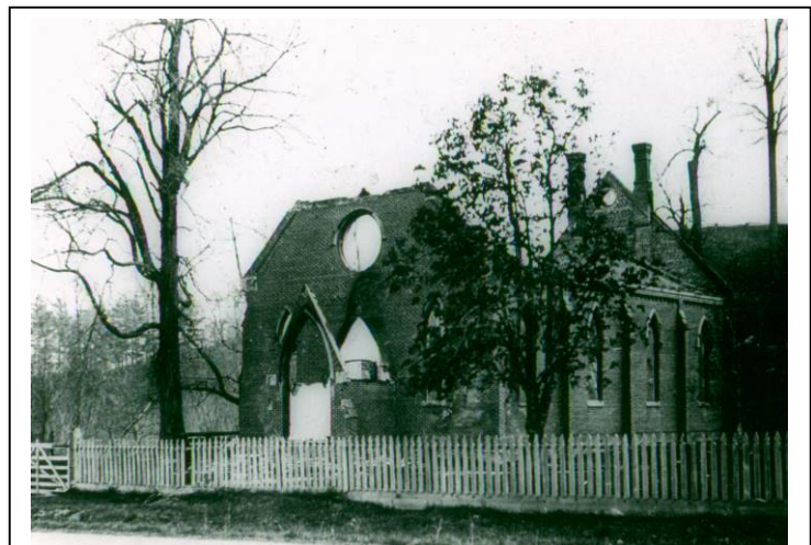
Figure 3. Aftermath of 1902 fire. There are detail differences with the current building shown in Fig 1: rose window above porch and lancet windows flanking, 4 windows along nave rather than 3, and more stone detailing. Photo from Vaughan Archive.
