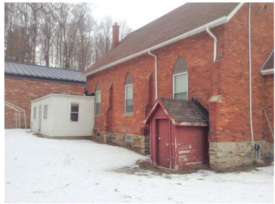
Figure 14. View from southeast.
