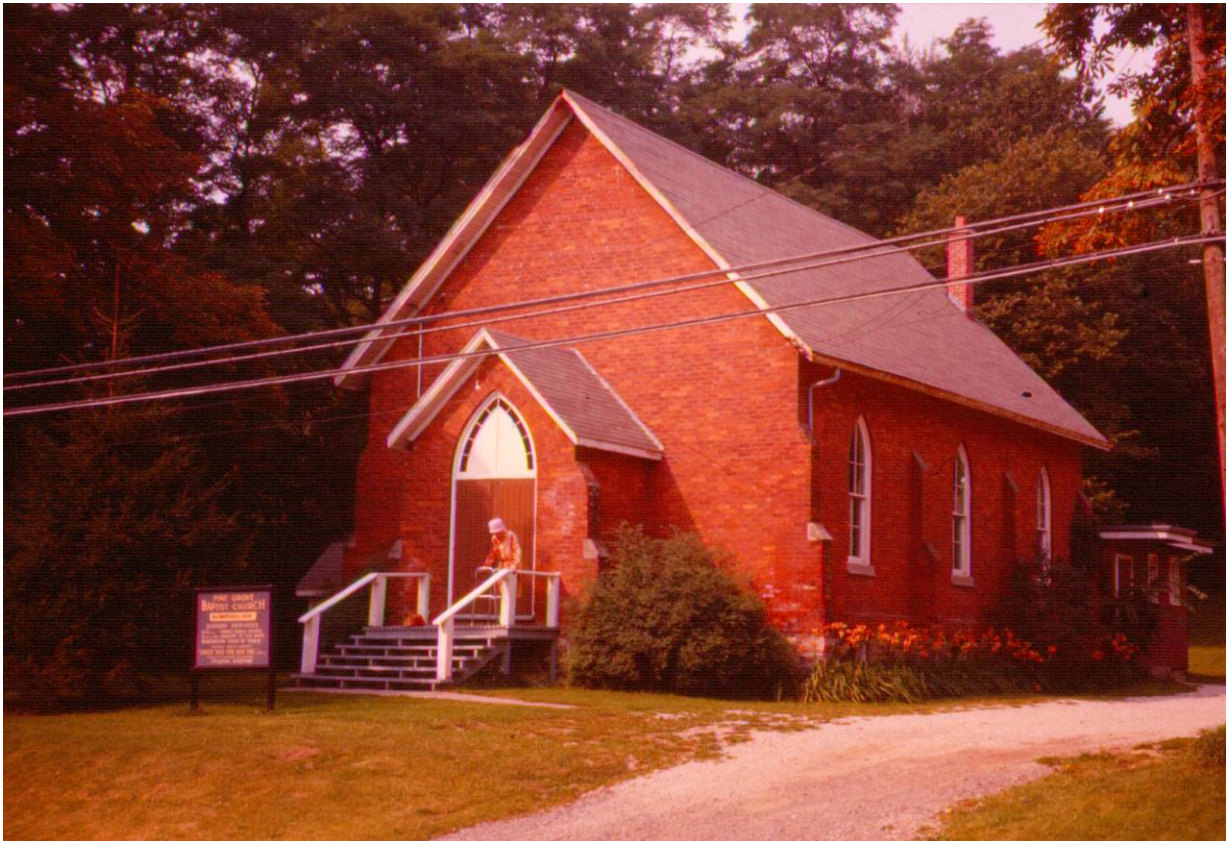
Figure 1. View from northeast, as Pine Grove Baptist Church in August, 1976. Photo from Vaughan Archive.
