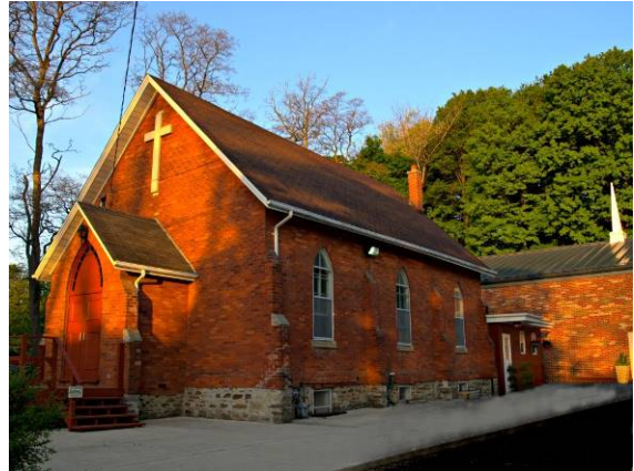
Figure 10. View from northeast, undated but post-2005. Photo by Mapio. Note that glazing fills entire lancet window openings.
