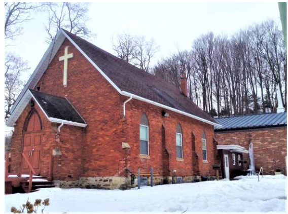
Figure 13. View from northeast. Note that pointed arches are now filled with plywood panels.
