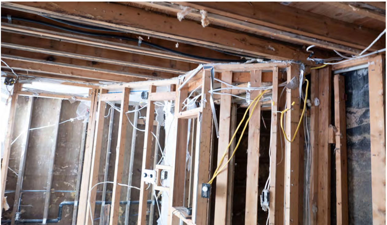
Figure 36: Moisture problems in the basement have resulted in the removal of previous finishes ( CBCollective, 2023 ).
