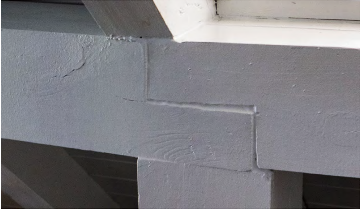
Figure 35: Use of filler shows lack of precision in joint ( CBCollective, 2023 ).
