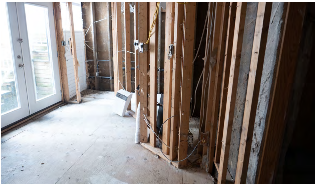
Figure 18: The rear addition in the basement, with plywood subfloor resting directly on grade (CBCollective, 2023).
