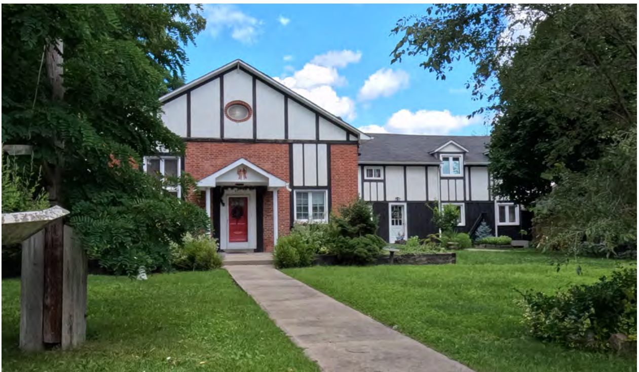
Figure 22: Looking north at 67 Napier Street. The brick building is c.1856 schoolhouse (note Flemish bond), and the half-timbered structure behind may also be historic. The c.1970 garage addition is out of frame to the right (CBCollective, 2023).
