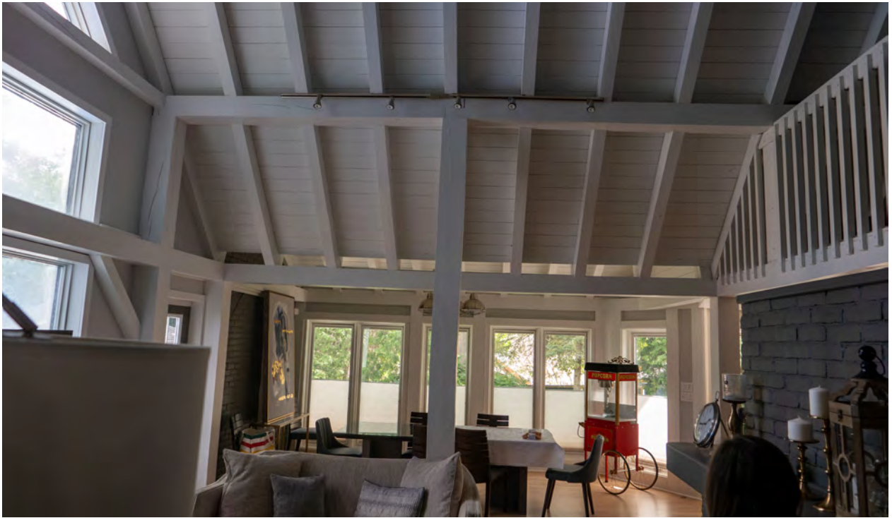
Figure 13: Exposed timbers in the north end living room (CBCollective, 2023).
