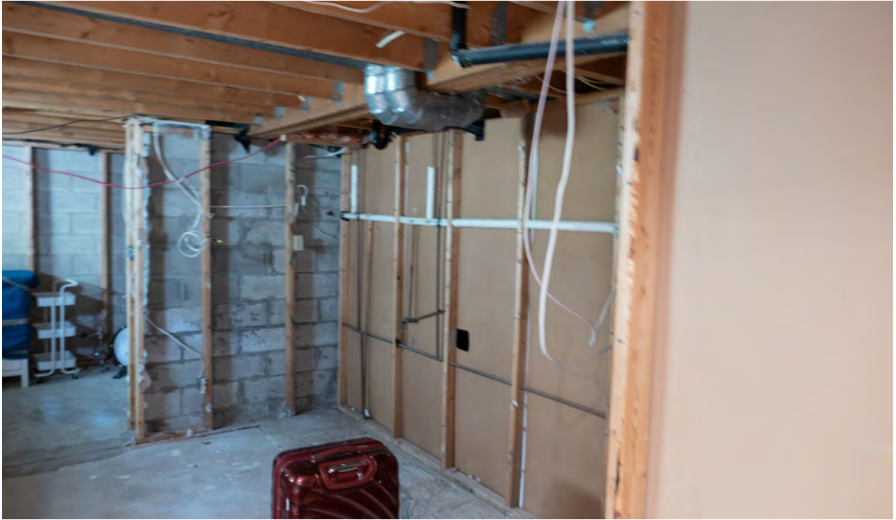
Figure 17: Modern framing and concrete block foundations in the basement (CBCollective, 2023).
