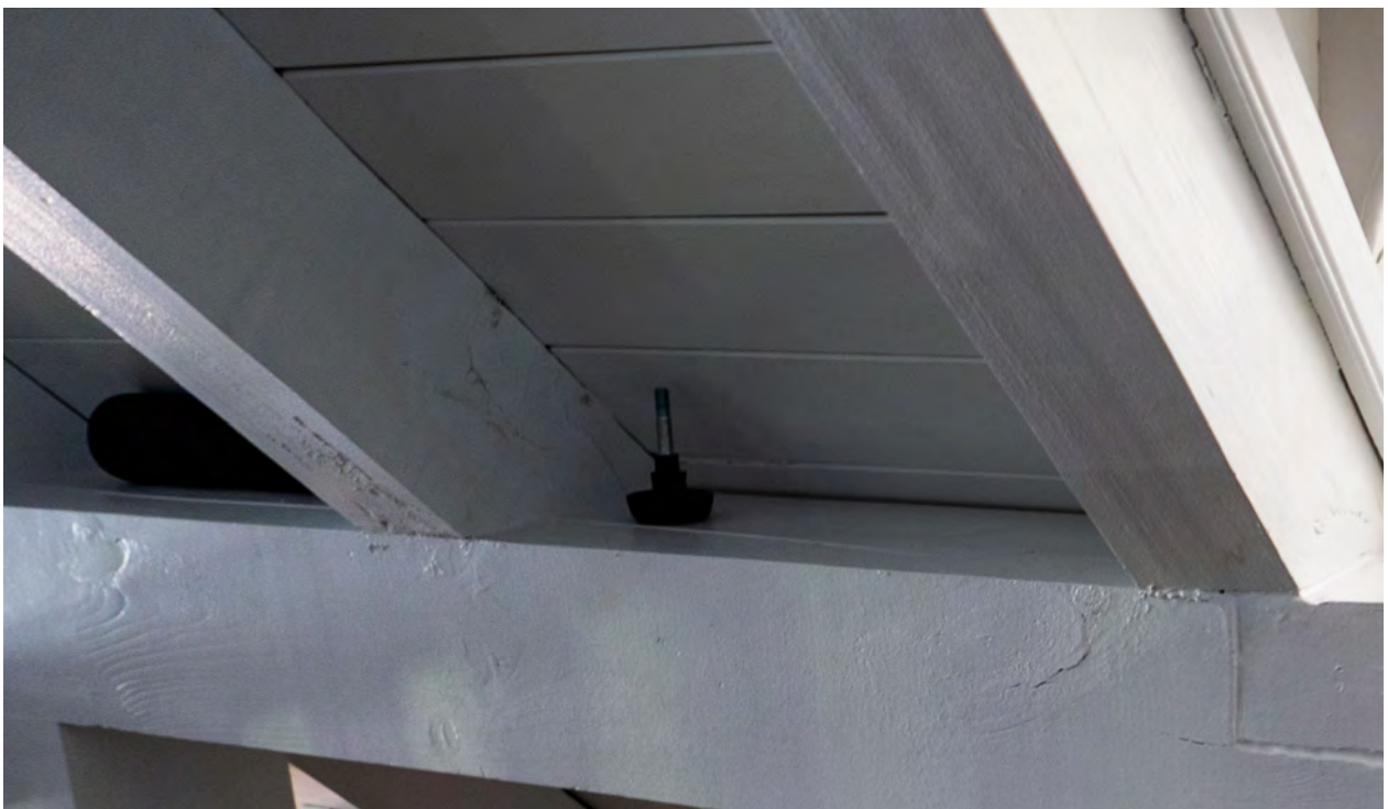
Figure 30: Timbers at 57 Napier Street do not show evidence of hand-tool finishing ( CBCollective, 2023 ).
