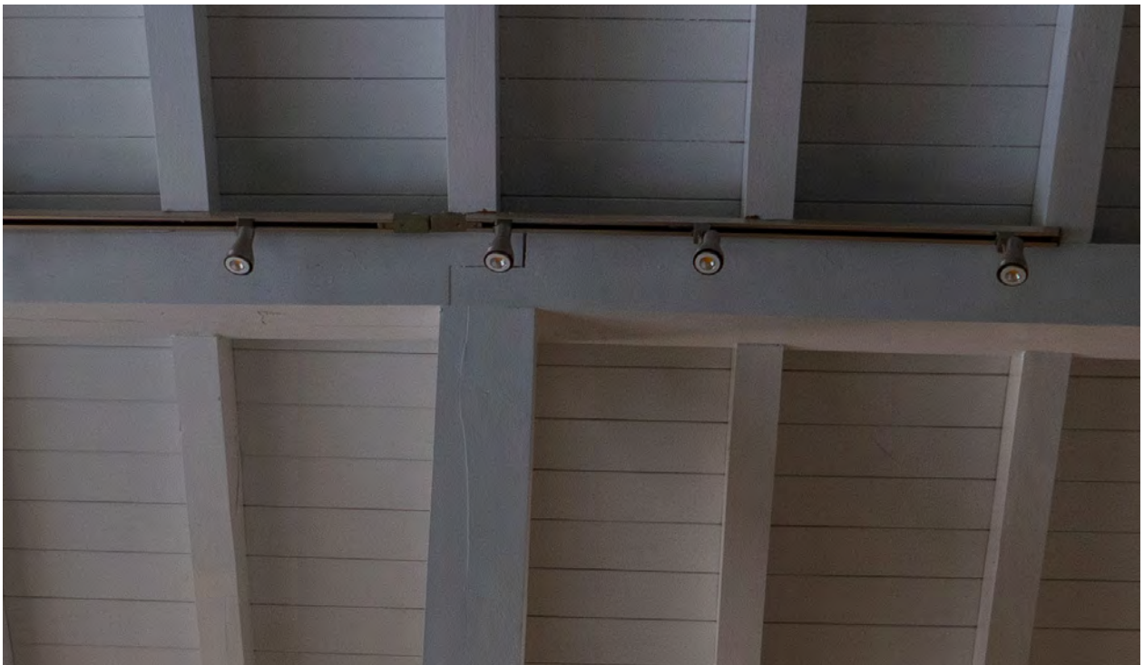
Figure 34: Joints are not particularly tight above the living room loft (CBCollective, 2023).
