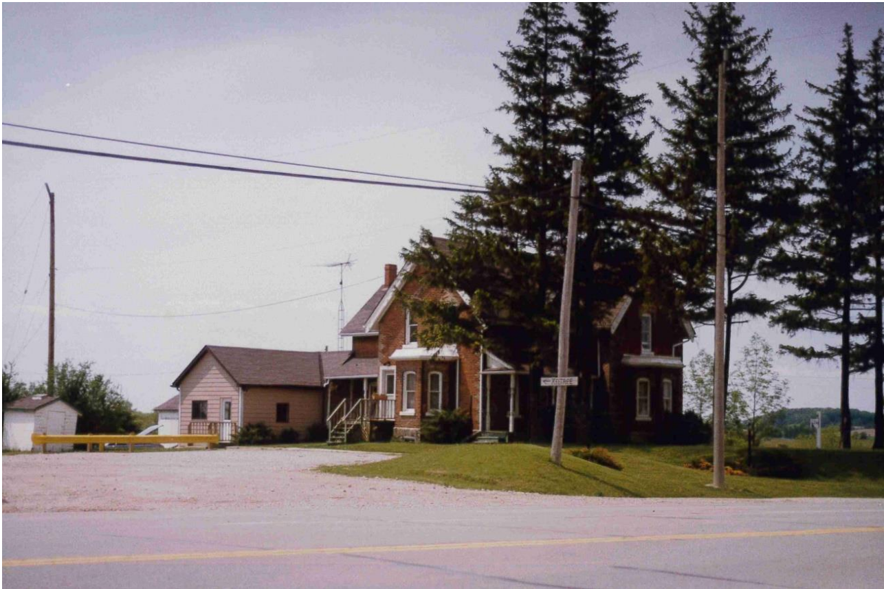
11244 Keele Street: South and east elevations, including view of addition, from Keele Street
