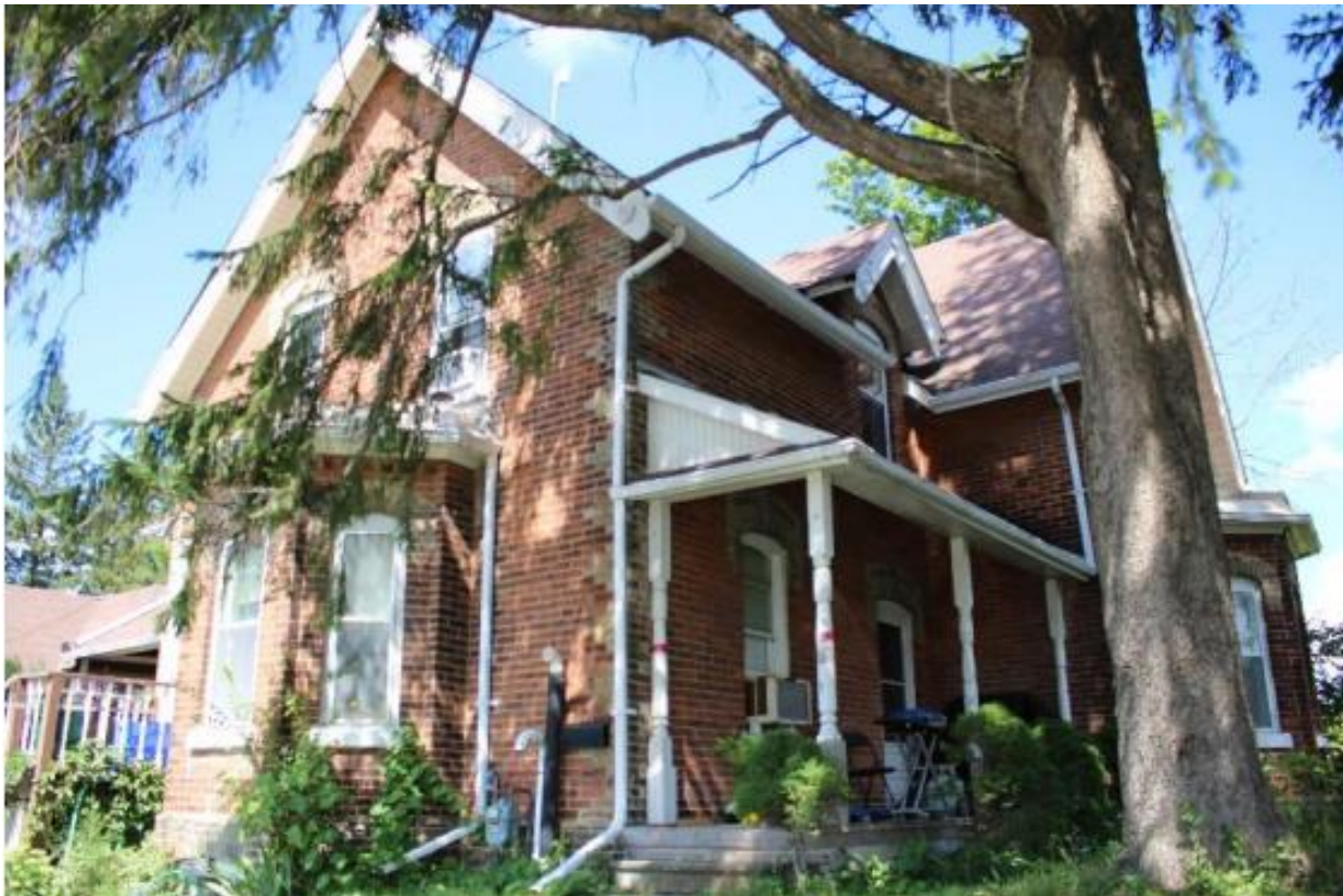
11244 Keele Street: South and east elevations (Source – Cultural Heritage Evaluation Report, A.S.I. 2022)
