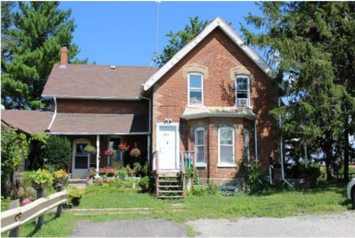
11244 Keele Street: South elevation (Source: Cultural Heritage Evaluation Report, A.S.I. 2022)
