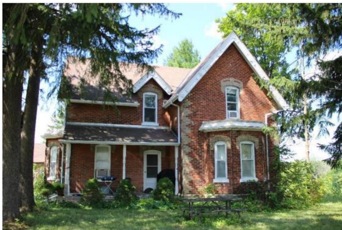
11244 Keele Street: East elevation, facing Keele Street (Source: Cultural Heritage Evaluation Report, A.S.I. 2022)
