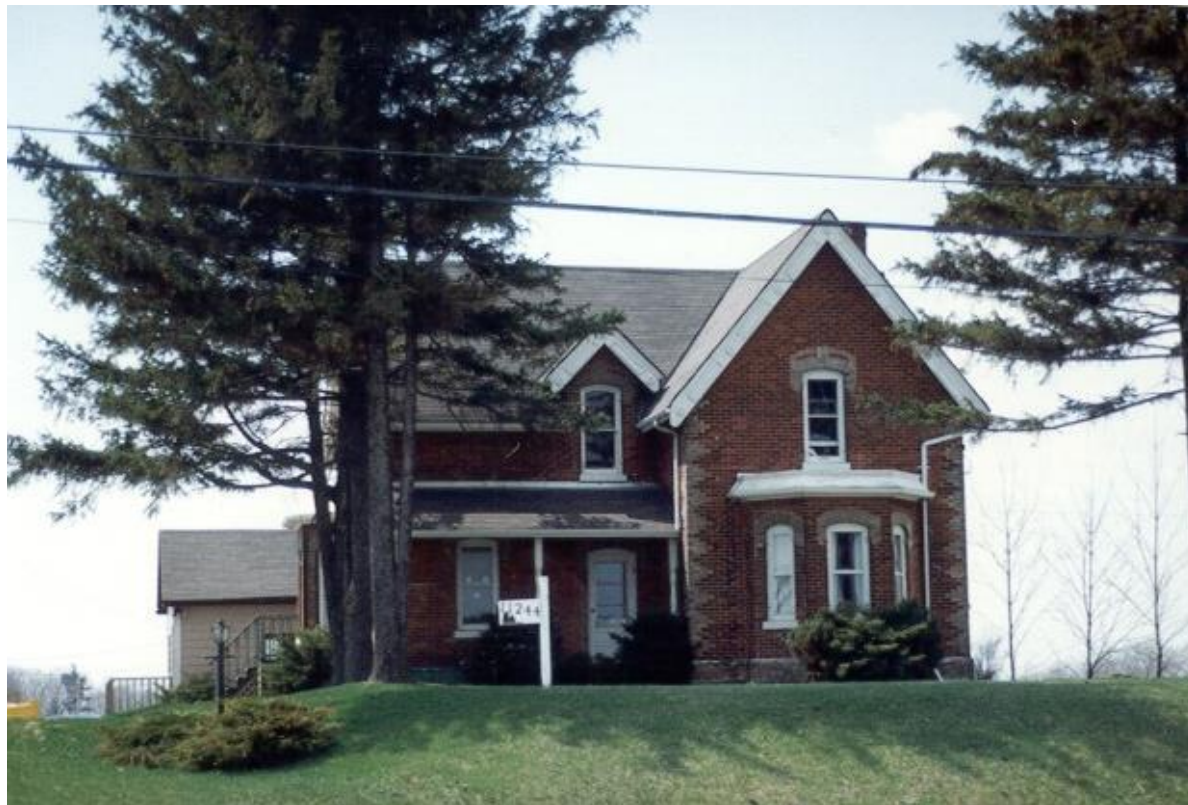
11244 Keele: East elevation, 2004 photo
