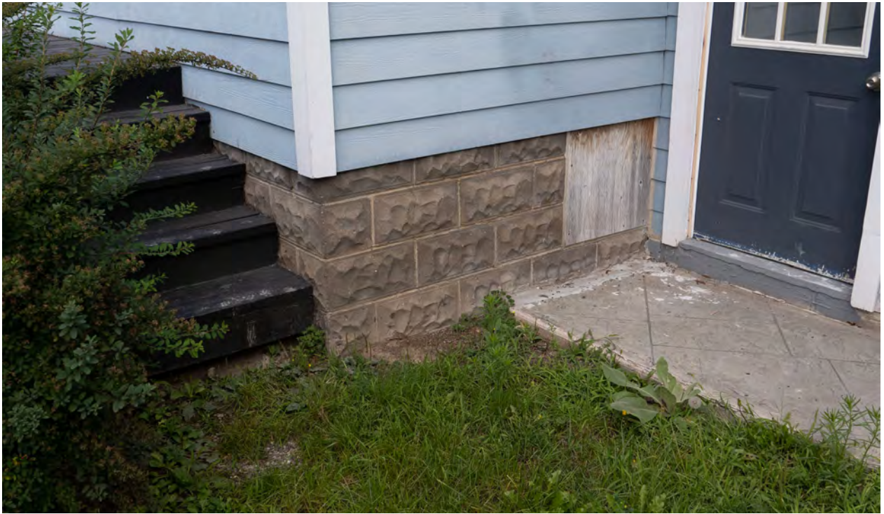
Figure 9: Remnants of the original cast foundation masonry, as seen at the rear (south) elevation (CBCollective, 2023).
