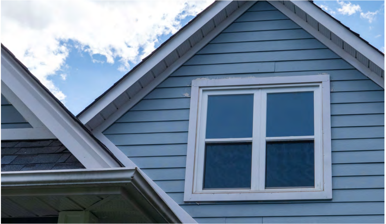
Figure 29: Paint failure noted around the window in the north gable (CBCollective, 2023).
