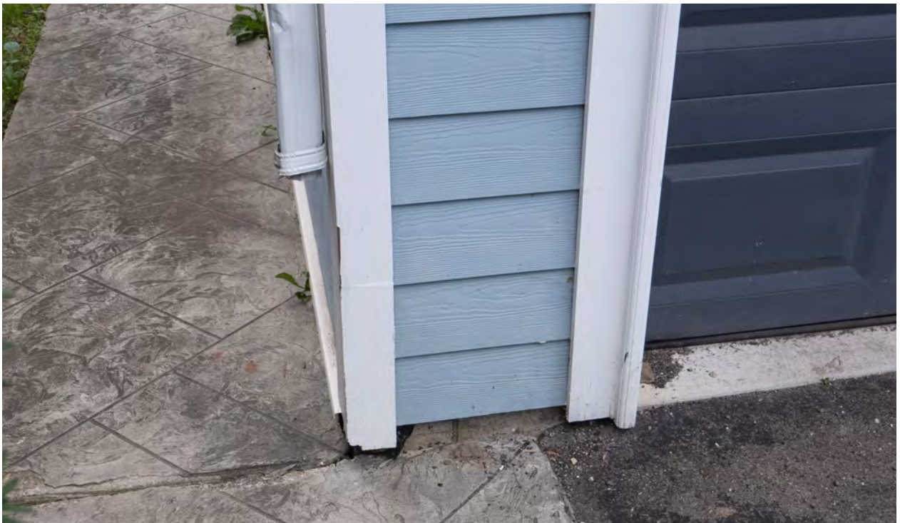
Figure 30: Minor rot observed at exposed end-grain boards on the garage addition, at the house's northeast corner (CBCollective, 2023).
