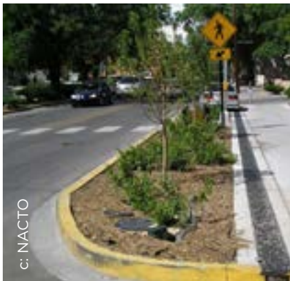
Figure 4.34. Mid-block curb extension.
