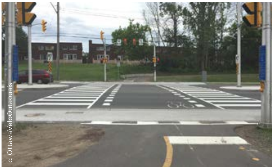
Figure 4.75. Mid-block crossside and bike signal for trail access.
