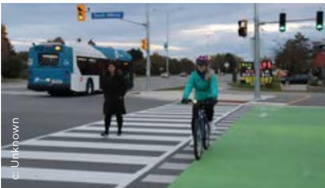
Figure 4.53. Crosswalk and crossside at major intersection.
