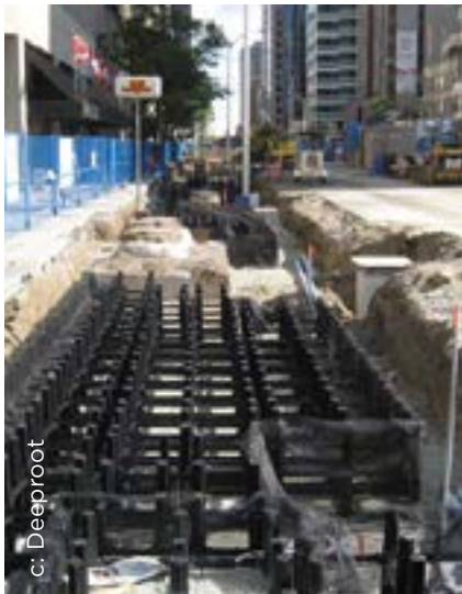
Figure 4.45. Soil cells (Bloor Street, Toronto).
