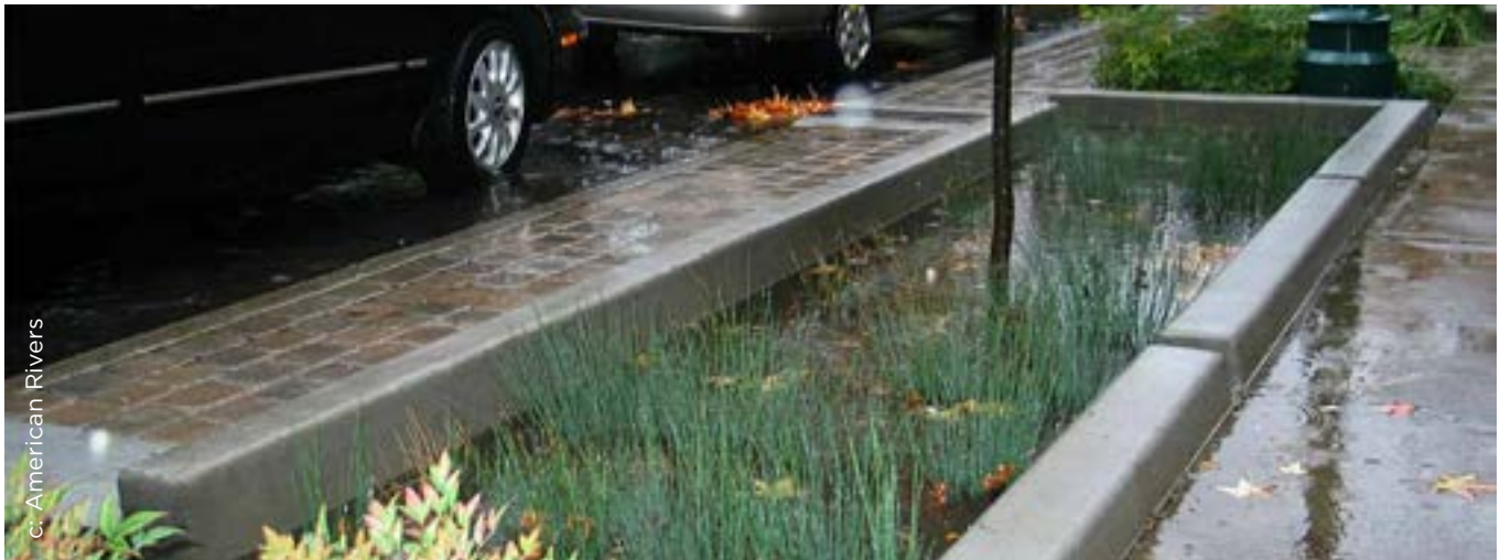
Figure 4.38. Stormwater management system: bioswale.
