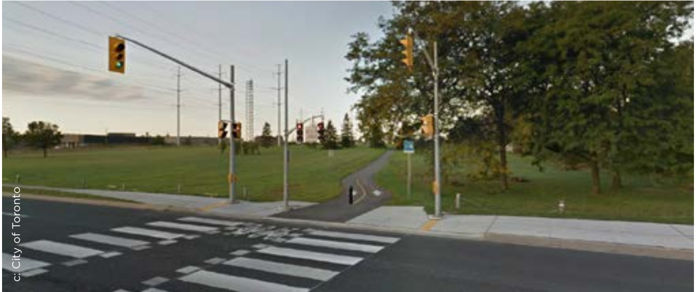
Figure 2.25. This image demonstrates how to consider the desire lines of trail users who want to cross a busy street. Providing a signalized junction with markings makes the connection more safe and convenient.
