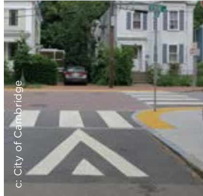
Figure 4.32. Raised crosswalk at intersection.
