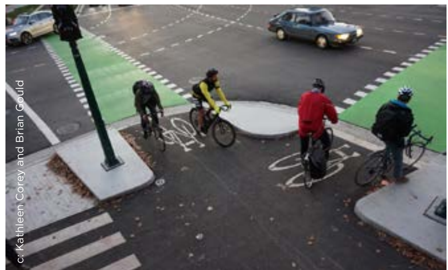
Figure 2.21. Protected intersections increase driver visibility of people in the crossbike and crosswalk by setting back the crossbike from the motor vehicle travel lane.
