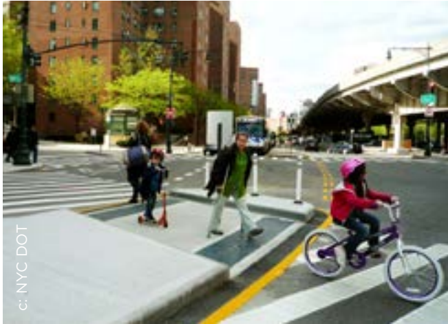
Figure 4.47. Accessible intersection for users of different ages and abilities.
