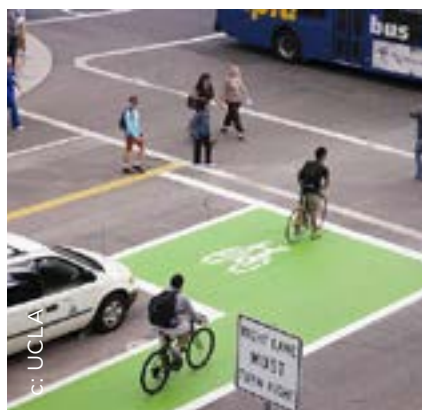
Figure 4.73. Bicycle box at signalized intersection.
