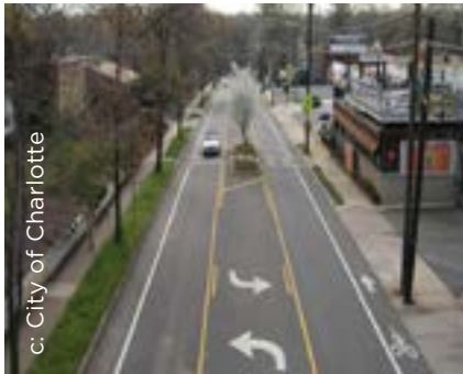
Figure 4.17. Lane reduction and conversion, addition of bike lanes, medians and pedestrian refuge islands.
