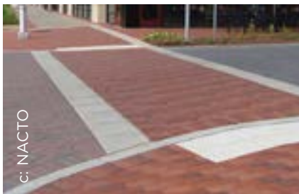
Figure 4.63. Raised driveway and the continuation of the paving material over the driveway highlights crossing of different users.
