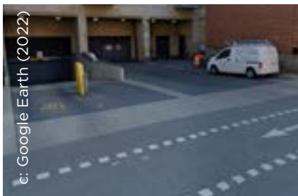
Figure 4.62. Raised driveway into parking garage.
