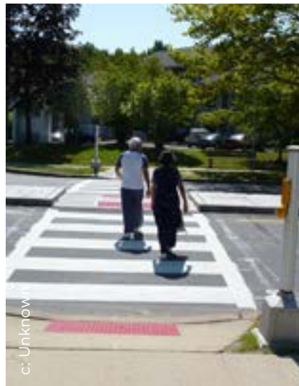
Figure 2.27. Mid-block crosswalks facilitate crossing along desire lines across streets to recreational trails, transit stops and schools.
