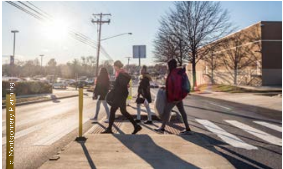
Figure 4.68. Pedestrian refuge with vertical elements and signage.
