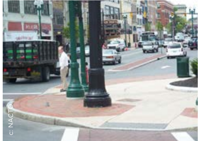
Figure 4.48. Compact corner radii at intersection.
