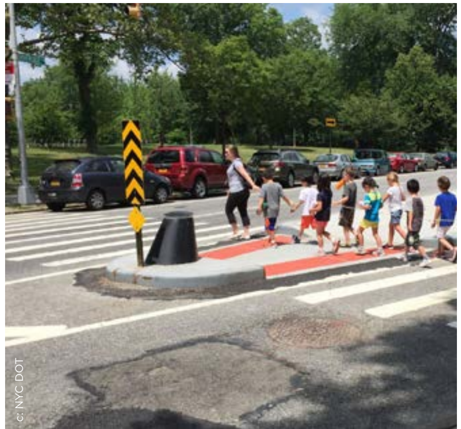
Figure 4.67. Pedestrian refuge island.
