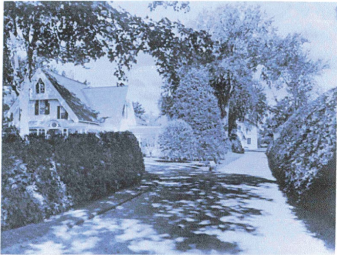
ENTRANCE TO DON HEAD HOUSE
