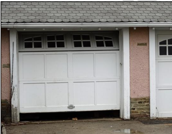
Figure 13: West façade of garage, 2016
