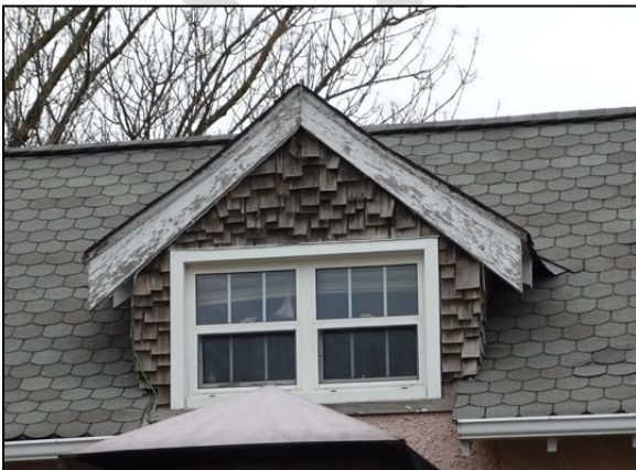
Figure 14: West gable with replacement shake cladding; roof with replacement asphalt cladding, 2016
