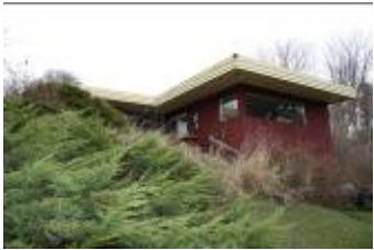
East Elevation of Kitchen
