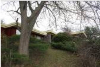
East Side: showing 1950's addition and kitchen addition
