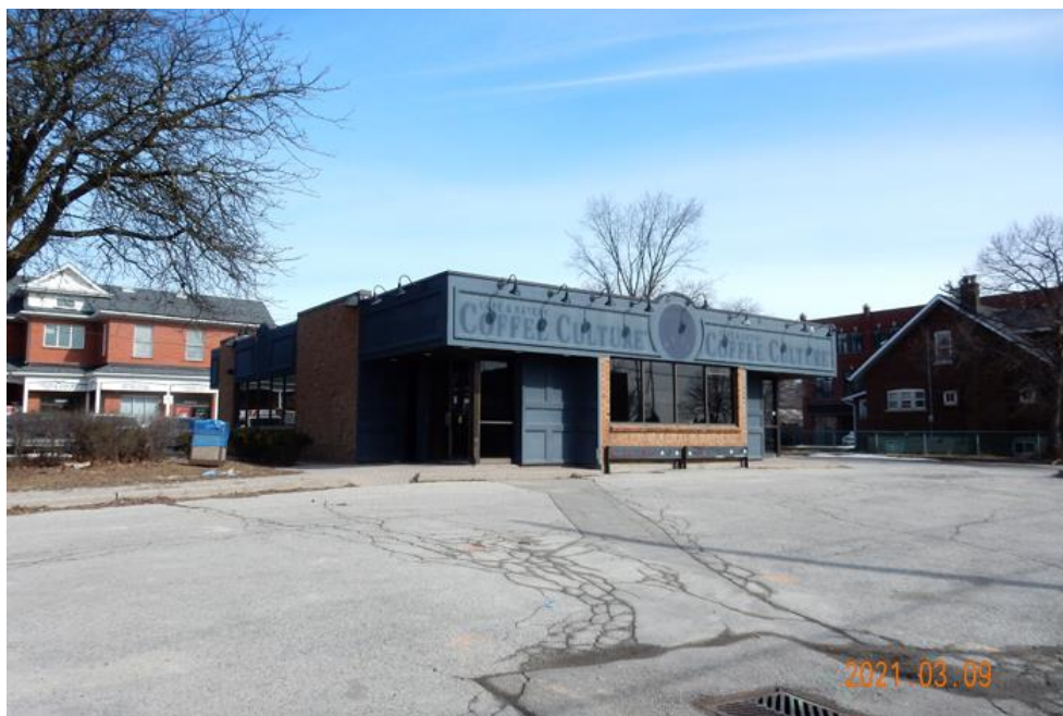
Figure 4: 10037 Keele Street Looking Northeast from Keele Street, LDW
