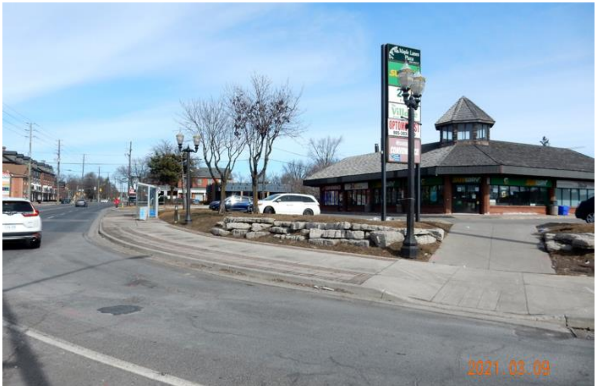
Figure 47: Plaza, Northeast Corner of Major Mackenzie Drive and Keele Street, LDW
