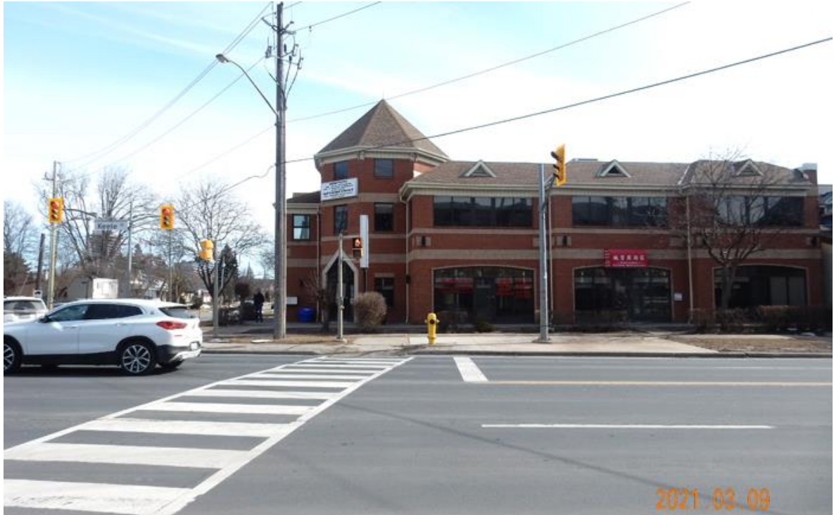
Figure 57: 10065 Keele Street - East Side - Southeast Corner of Keele and Railway Streets, LDW
