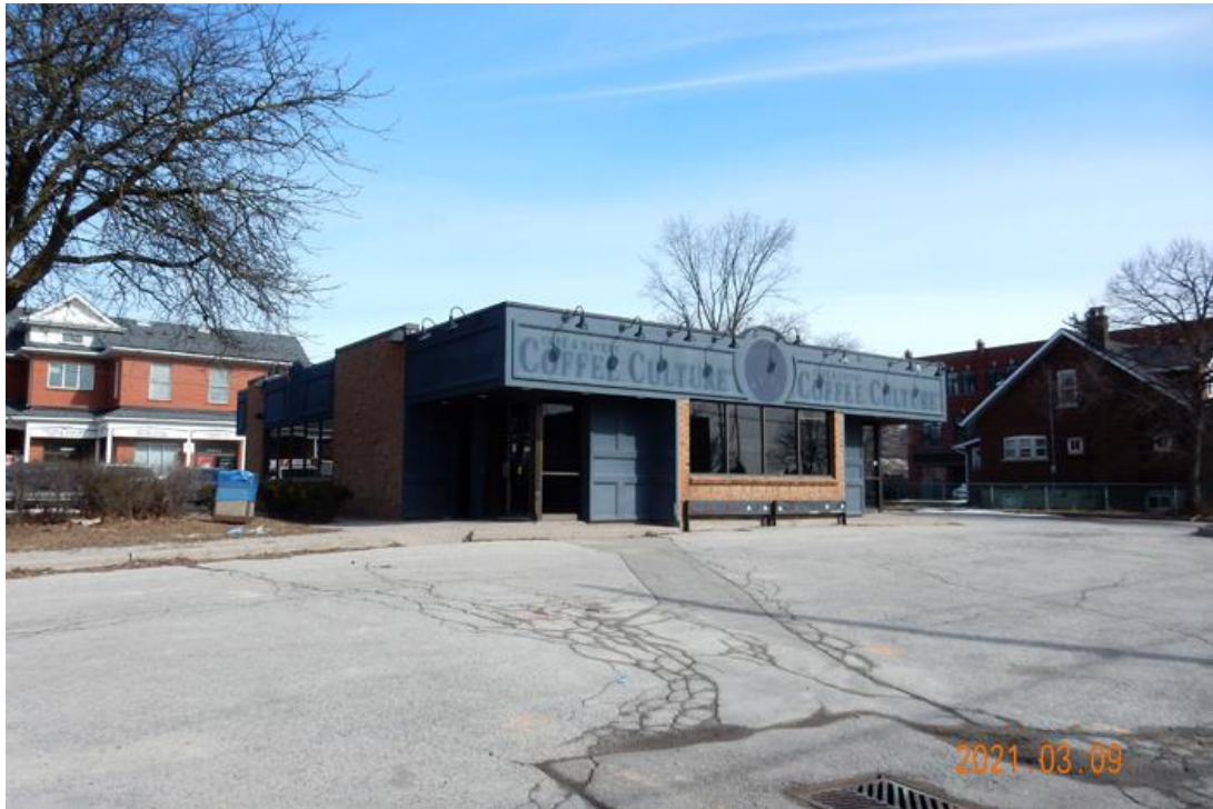
Figure 38: 10037 Keele Street Looking Northeast from Keele Street, LDW
