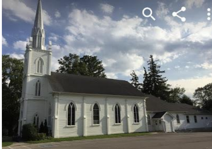
Figure 19: St. Andrews Presbyterian Church, Google Maps
