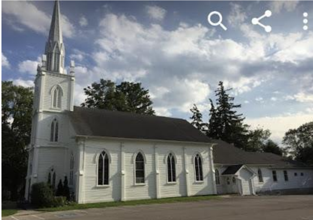
Figure 45: St. Andrews Presbyterian Church, Google Maps
