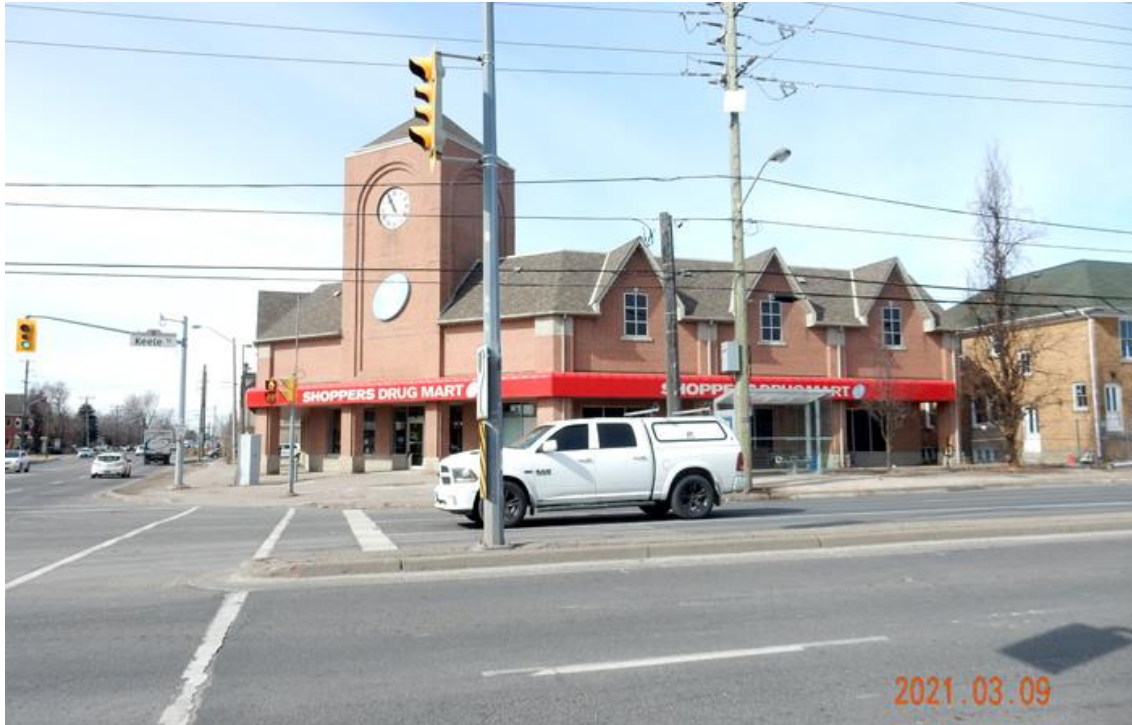
Figure 48: Shoppers Drug Mart, Northwest Corner of Major Mackenzie Drive and Keele Street, LDW
