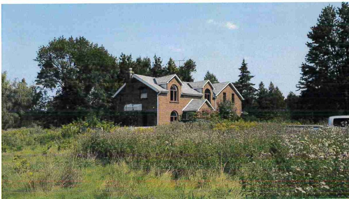
Figure 26: West end wall and south façade.
