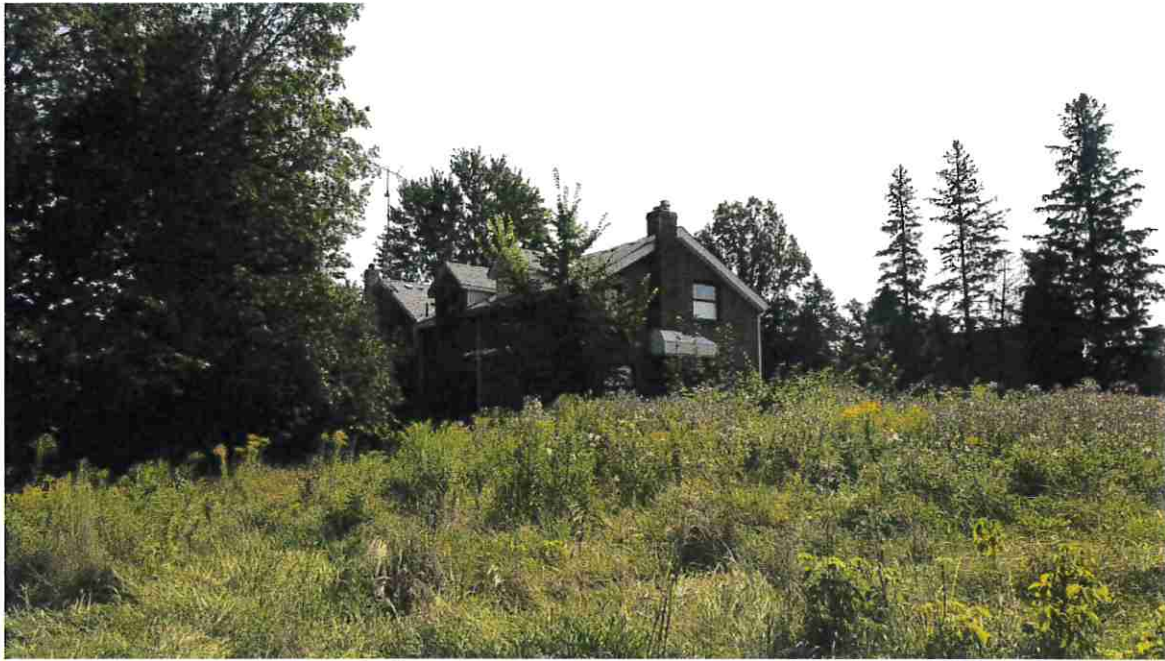
Figure 24: North façade and west end wall.
