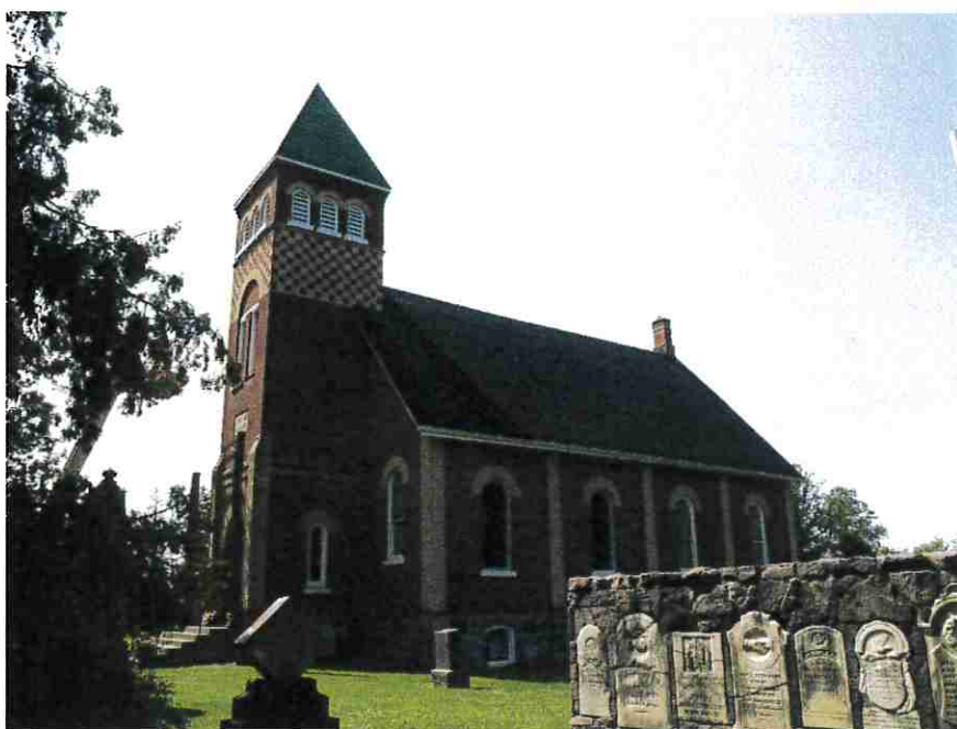
Figure 18: East and north façades.
