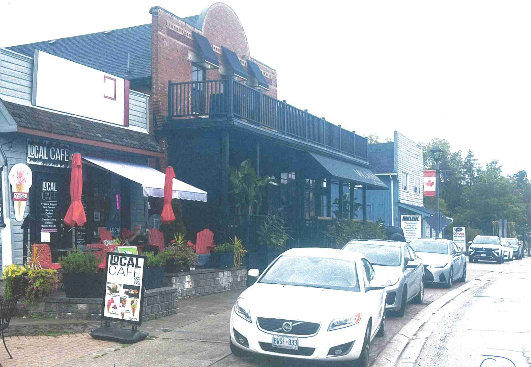
HERITAGE BUILDINGS (EAST SIDE)
