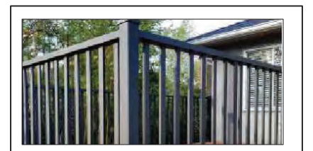
11. Exterior Metal Railing and Guards
