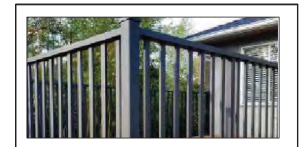
11. Exterior Metal Railing and Guards
