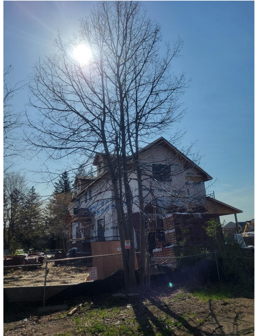
Photo 10. Tree 18, view looking southeast
