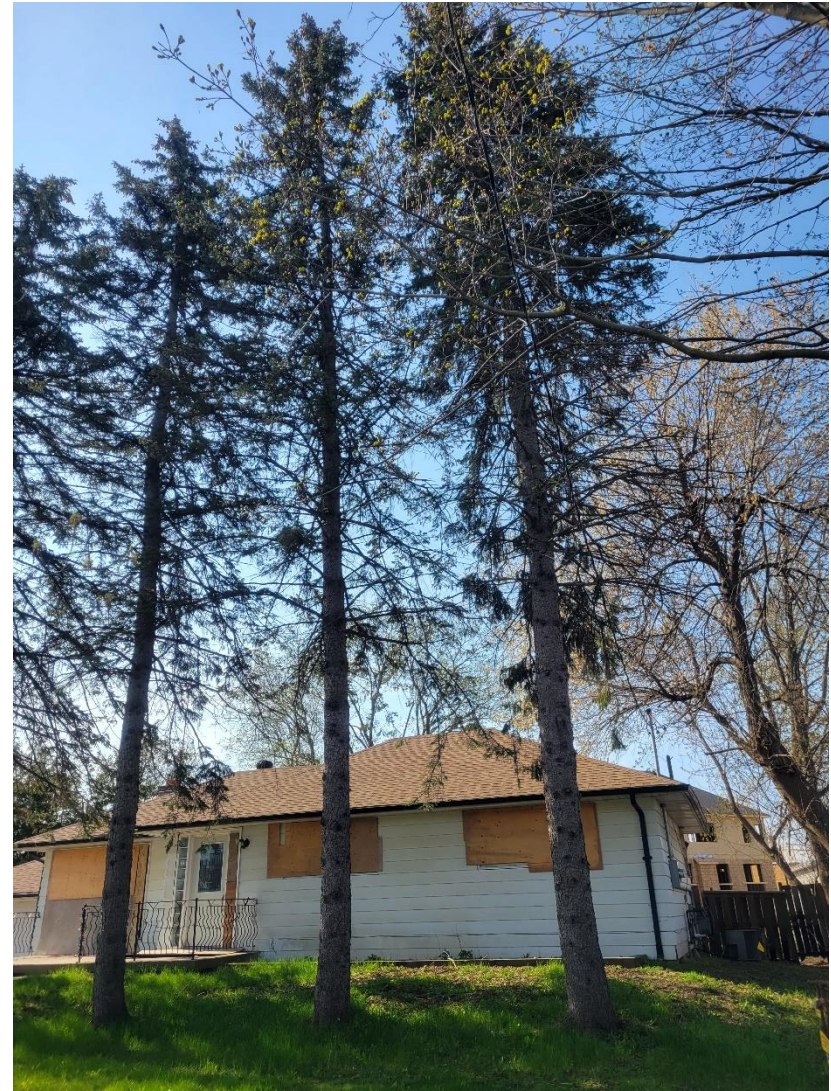
Photo 6. Trees 10 to 12, view looking southeast
