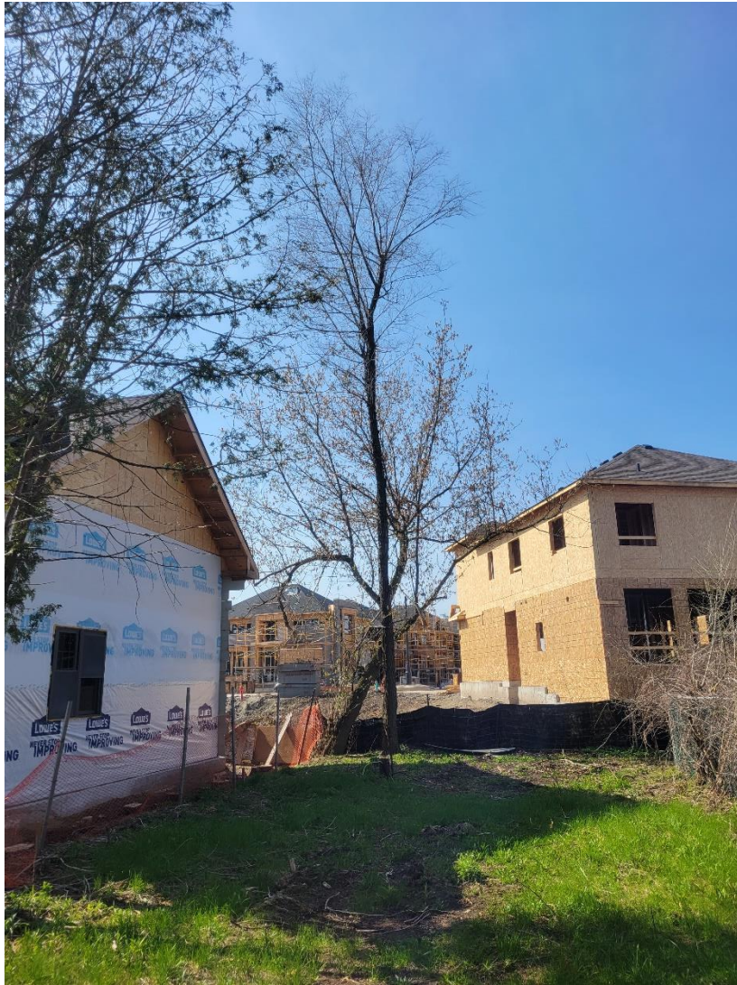
Photo 13. Trees 20 and 21, view looking southeast
