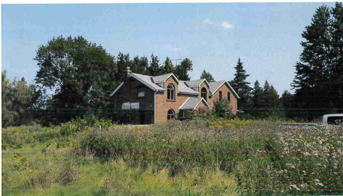
Figure 26: West end wall and south façade.
