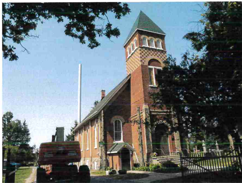
Figure 15: South and east façades of St. Paul's Presbyterian Church.
