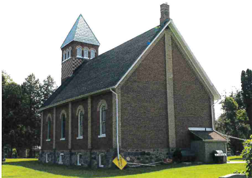
Figure 17: North façade and west end wall.
