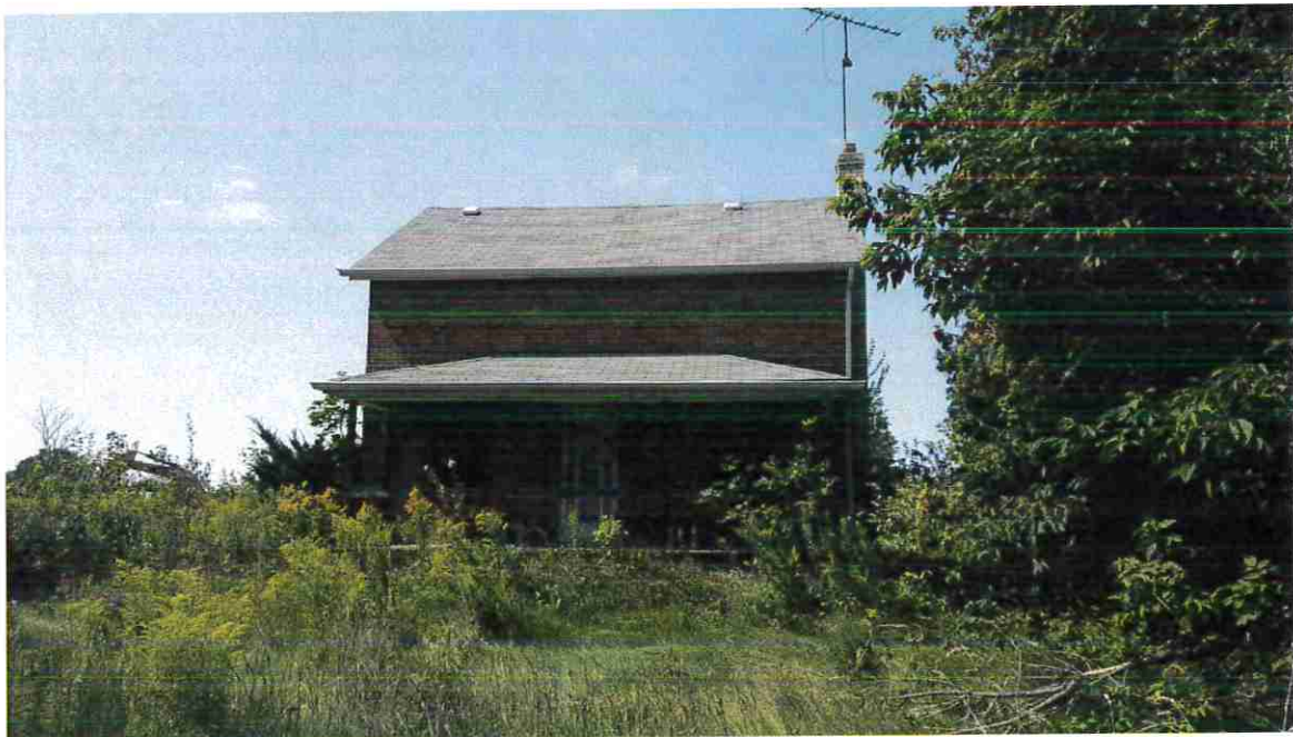
Figure 23: East or principal façade of the Caretaker's House.
