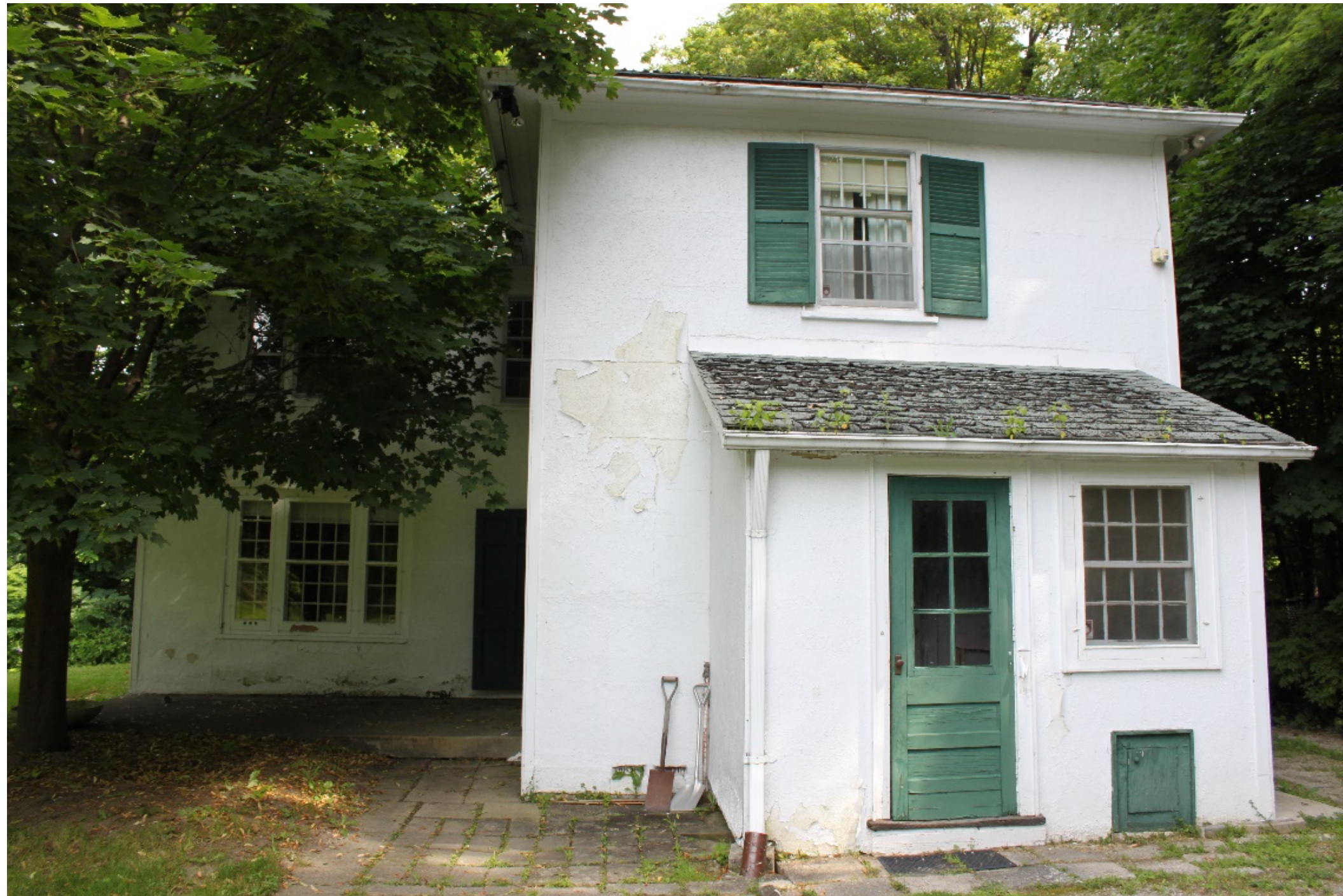
141 Centre Street – South Elevation – staff photo 2011
