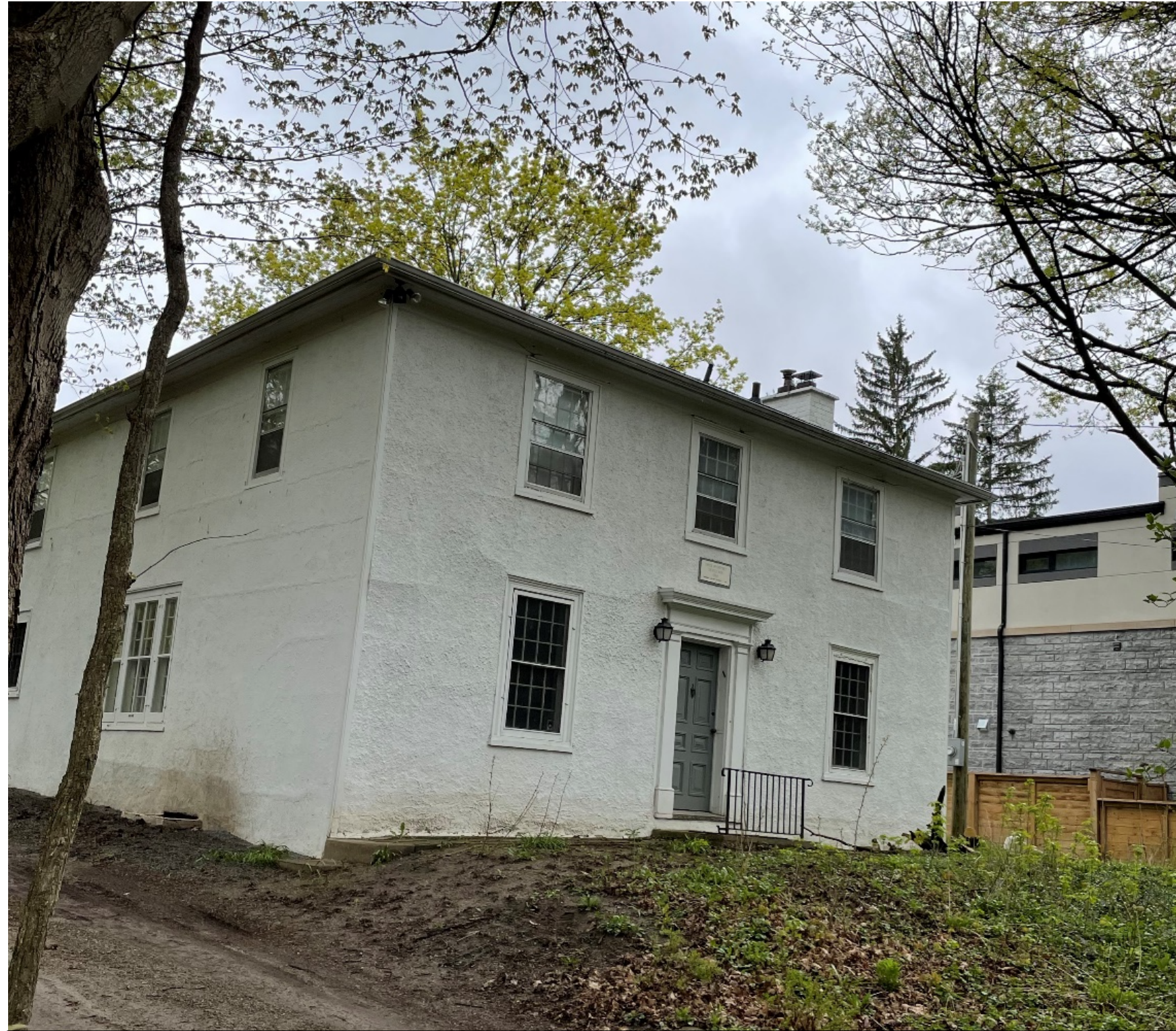
141 Centre Street – North and East Elevation – staff photo 2023
