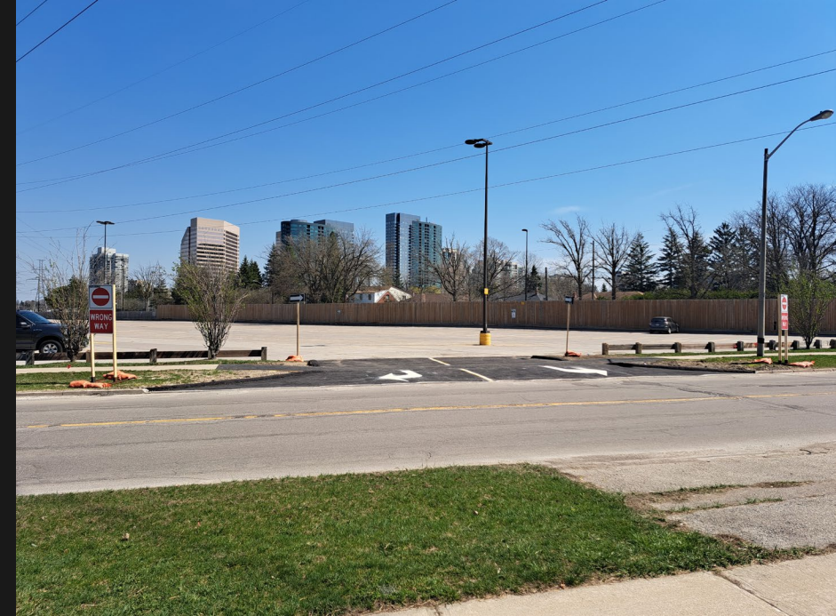
Excavation work around utility and TTC underground structures (Top) and Completed Talbot Road Temporary Exit (Bottom)
