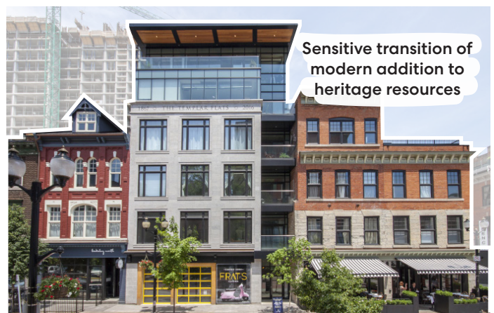
Figure 31. Templar Flats in Hamilton source: Ontario Association of Architects
