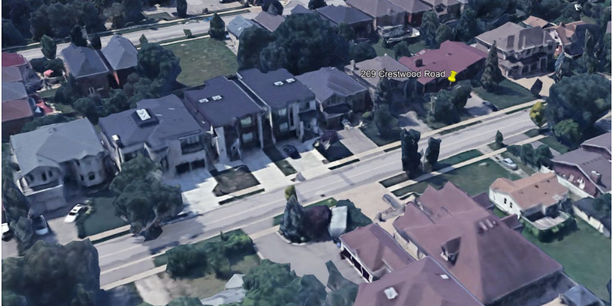
Figure 1 – 195 to 211 Crestwood Road (Source: Google Streetview)
