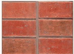
Precast unit pavers on concrete base
