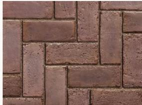
Precast unit pavers on concrete base
