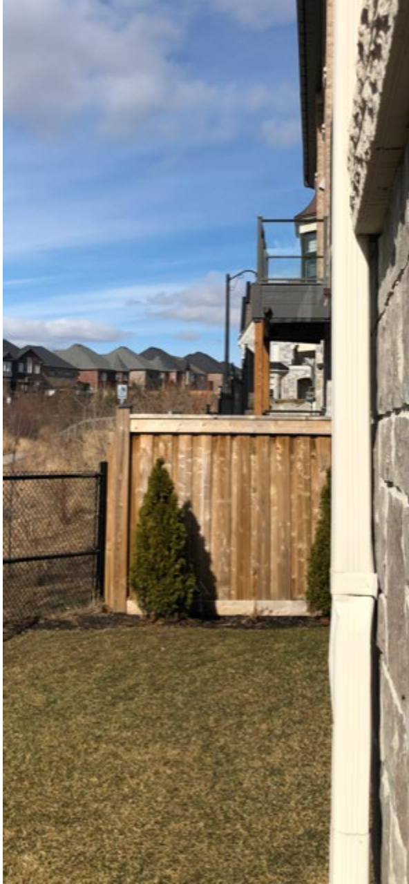
Illustration of decreased privacy (visual intrusion) on the side of our house as a result of the side deck
