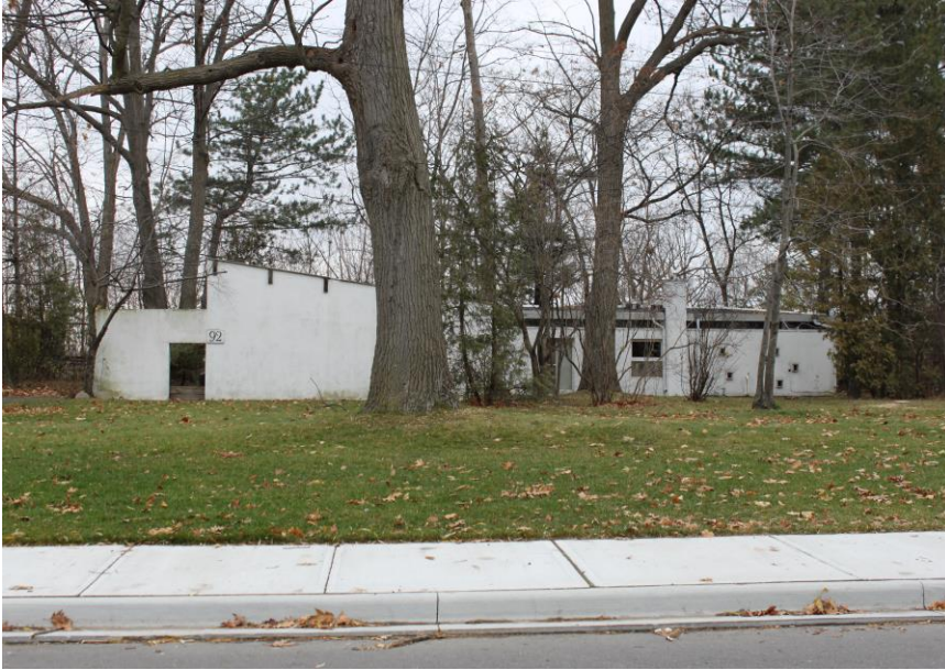
Fig. 23 Building at 92 Monsheen Drive., designed by architect Jerome Markson.
