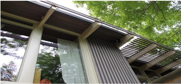
Fig. 42. Sun shade feature over rear deck, length of façade, 82 Monsheen Drive.
