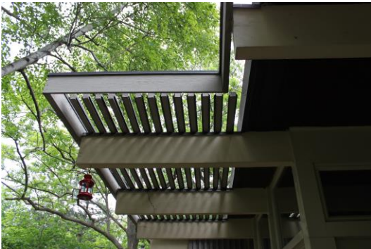
Fig. 43. Sun shade over rear façade and deck, 82 Monsheen Drive.
