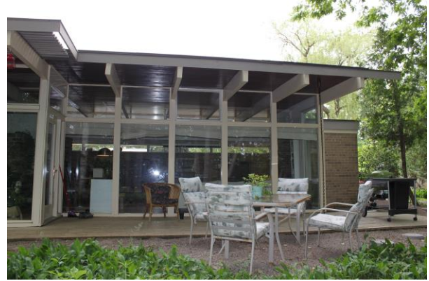
Fig. 17. West View of Living Room glazed wall. Barclay House, 82 Monsheen Drive, Woodbridge. Photo by Cultural Services, June 2011.
