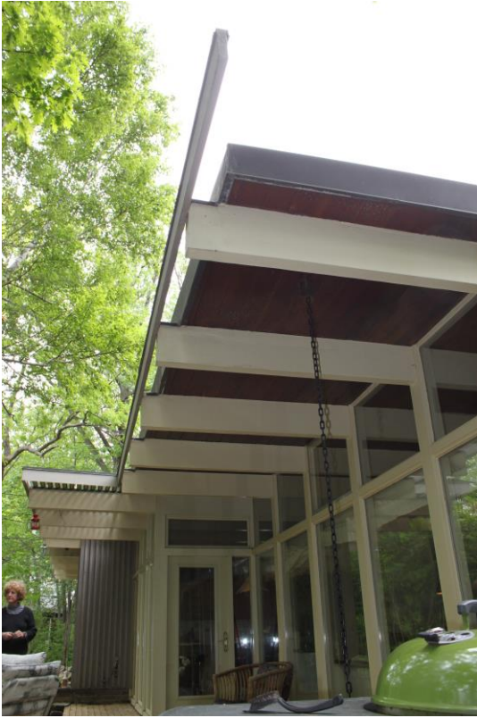
Fig. 41. Exterior beam transition to rear deck, 82 Monsheen Drive.
