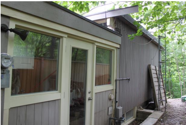
Fig. 20. North side yard and elevation view showing main portion of house. Barclay House, 82 Monsheen Drive, Woodbridge. Photo by Cultural Services, June 2011.
