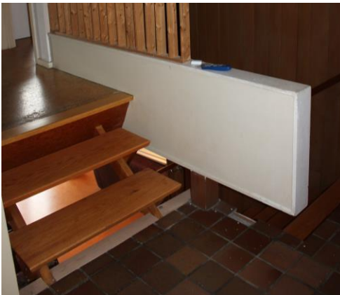
Fig. 35. Wood stairs transition from main living area to bedroom and den area. Also shown: interior clay (Ruabon) tile and cork tile flooring.
