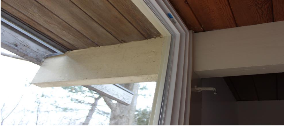
Fig. 34. Transition of open beam from interior to exterior, 82 Monsheen Drive.
