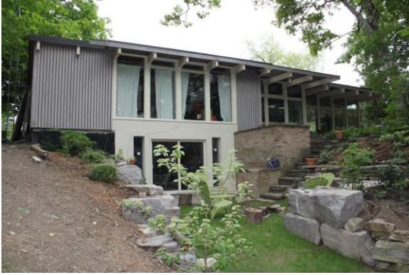
Fig. 16. West View. Barclay House, 82 Monsheen Drive, Woodbridge. Photo by Cultural Services, June 2011.
