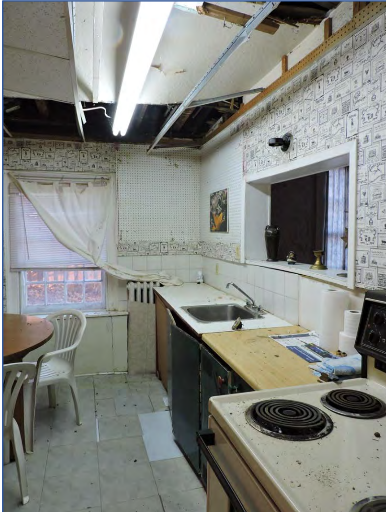
Figure 33: Kitchen located on main floor
