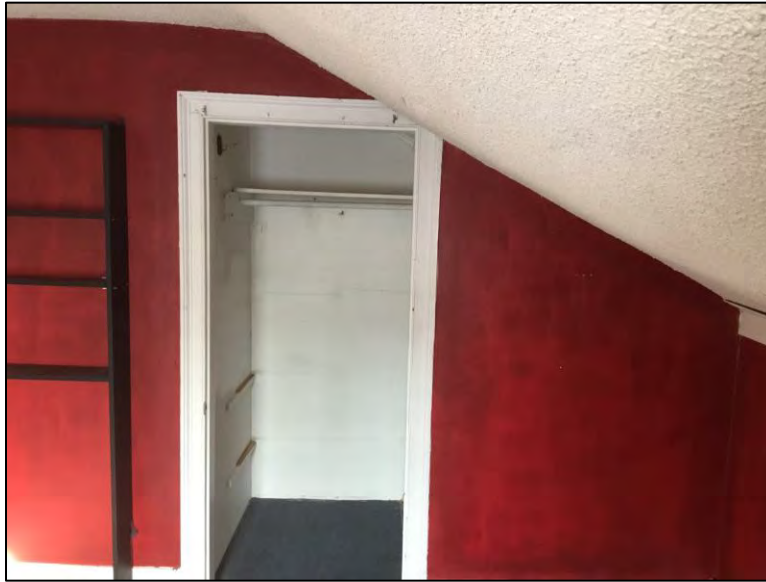
Photograph 1: Second-storey ceiling on east elevation
