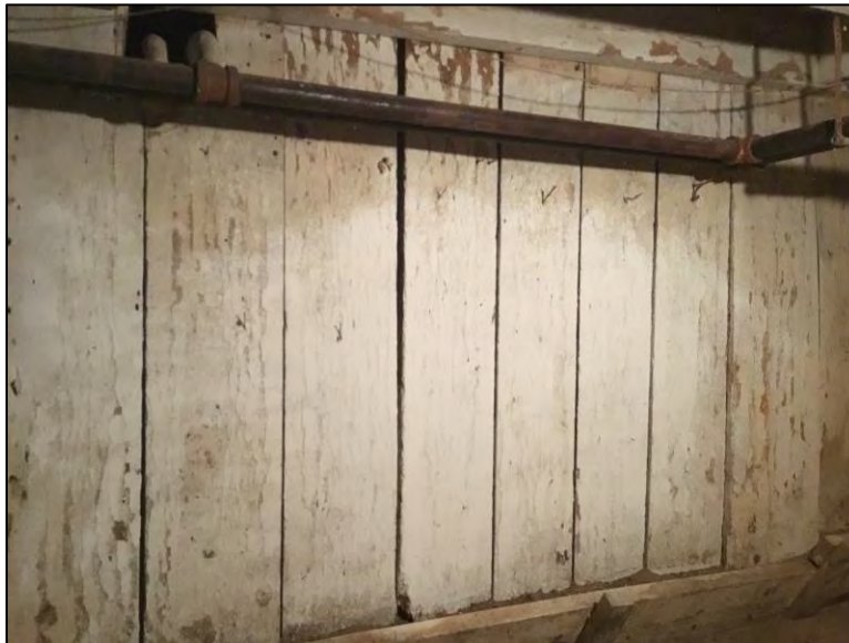
Photograph 6: Wood slat shoring
