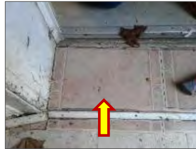
Photo 13: Non-asbestos 12" x 12" pink vinyl floor tiles in the Back Entrance (Loc. 2).
