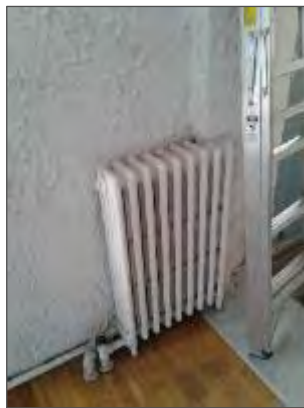
Photo 5: Uninsulated radiator in the Living Room and Dining Room (Loc. 4).
