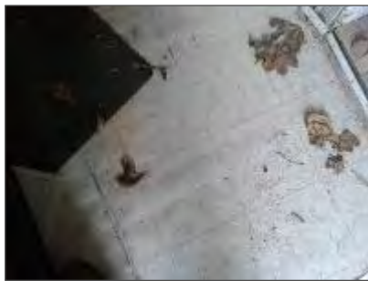
Photo 10: Non-asbestos pink vinyl sheet flooring on the floor of the Back Entrance (Loc. 2).
