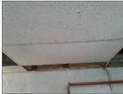
Photo 7: Non-asbestos 24" x 48" lay-in, fissure and pinhole ceiling tile in the Kitchen (Loc. 3).
