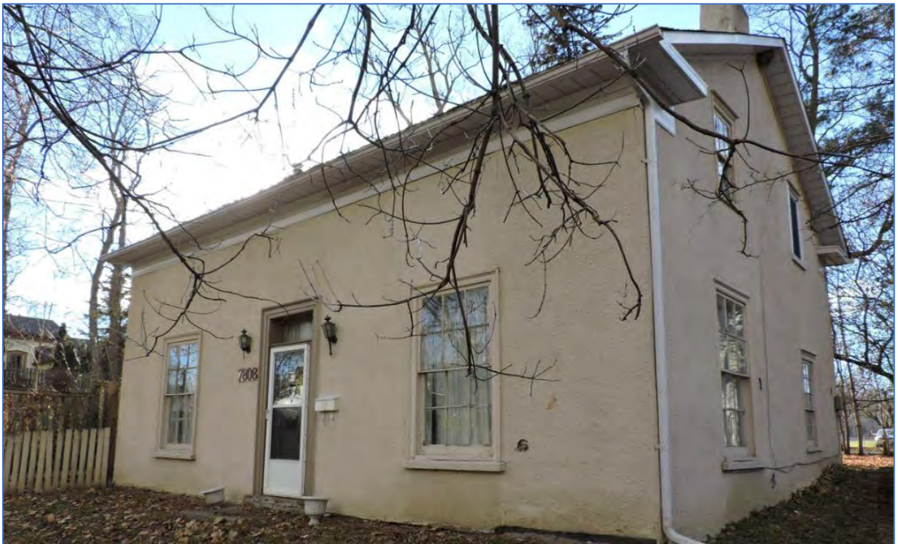
Figure 26: View southwest at the front façade and side elevation of the house on the Property
