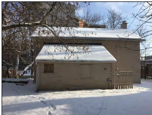
Photograph 9: Lean-to on west elevation
