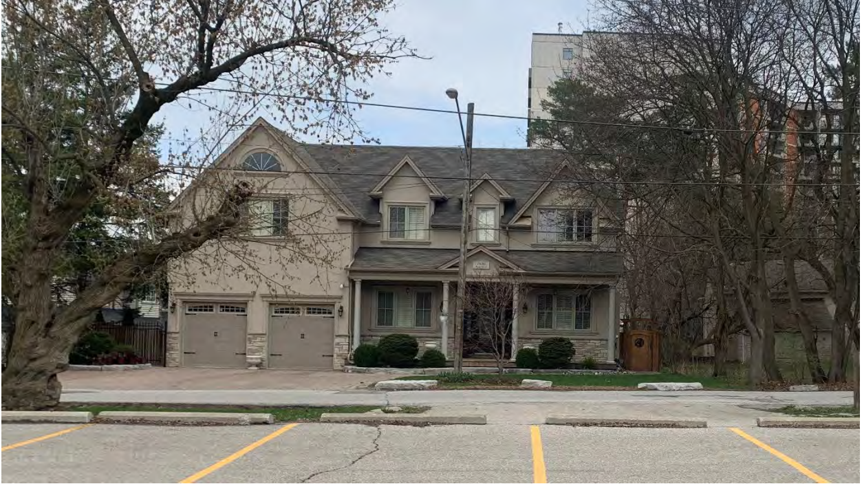
Figure 21: View east at the front of 7820 Yonge Street
