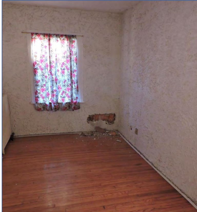
Figure 35: Study located on main level
