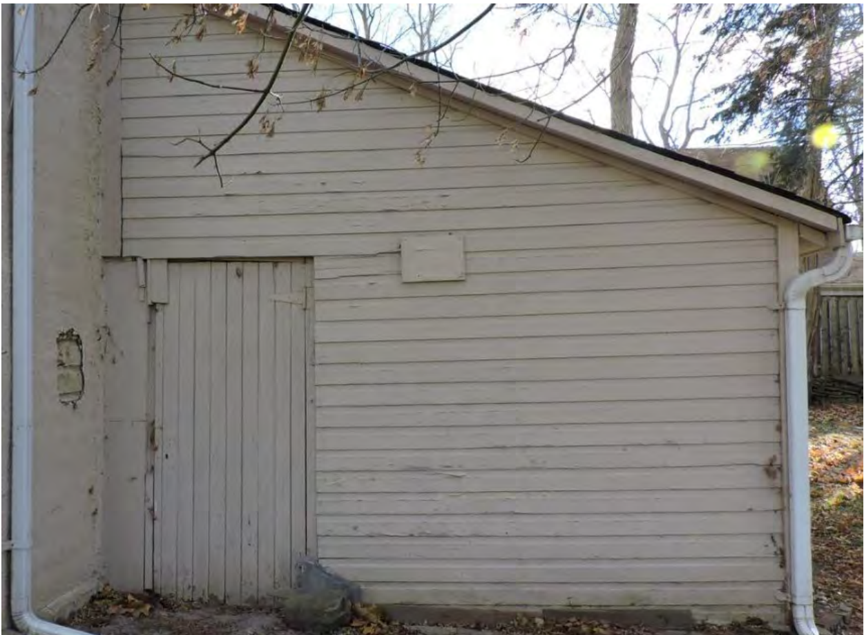
Figure 30: View south at the side of the rear lean-to-shed attached to the house on the Property
