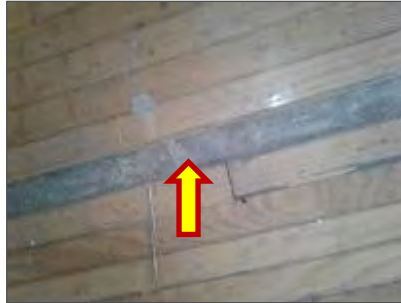
Photo 17: Non-asbestos beige paper below wood flooring in the Living Room and Dining Room (Loc. 4).
