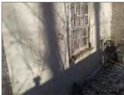
Photo 8: Non-asbestos plaster on the exterior walls (Loc. 8).
