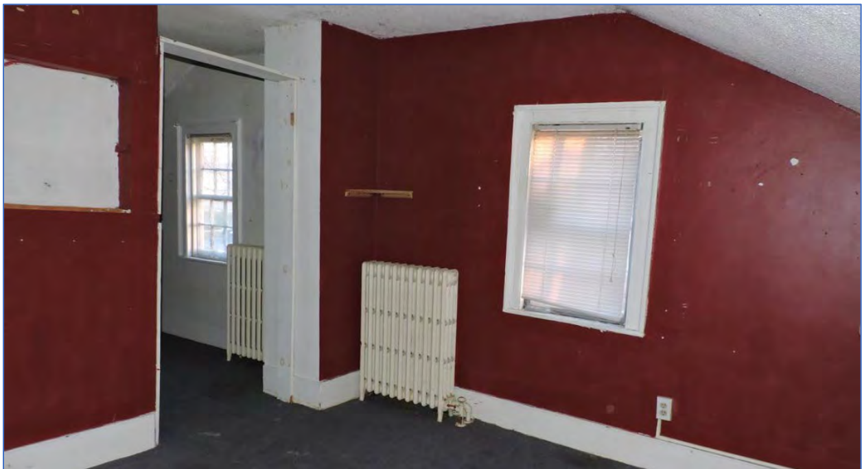
Figure 42: Bedrooms 2 and 3 on upper level
