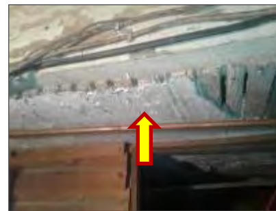
Photo 9: Non-asbestos plaster on the ceiling of the Basement (Loc. 7).
