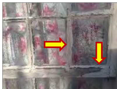
Photo 16: Non-asbestos beige caulking on exterior window frames.
