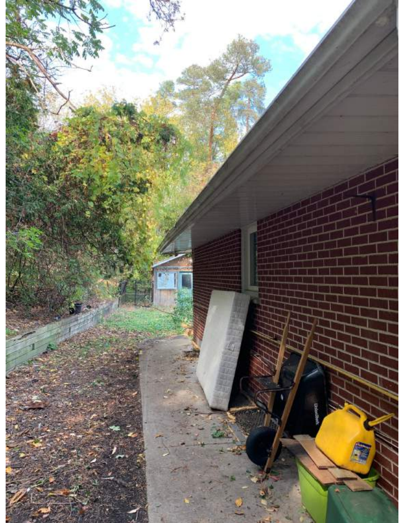
West elevation, view from south
