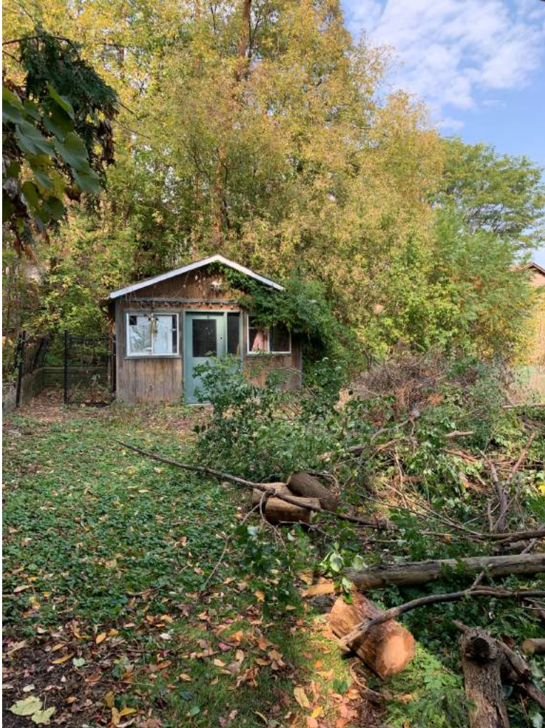
Shed, view from south
