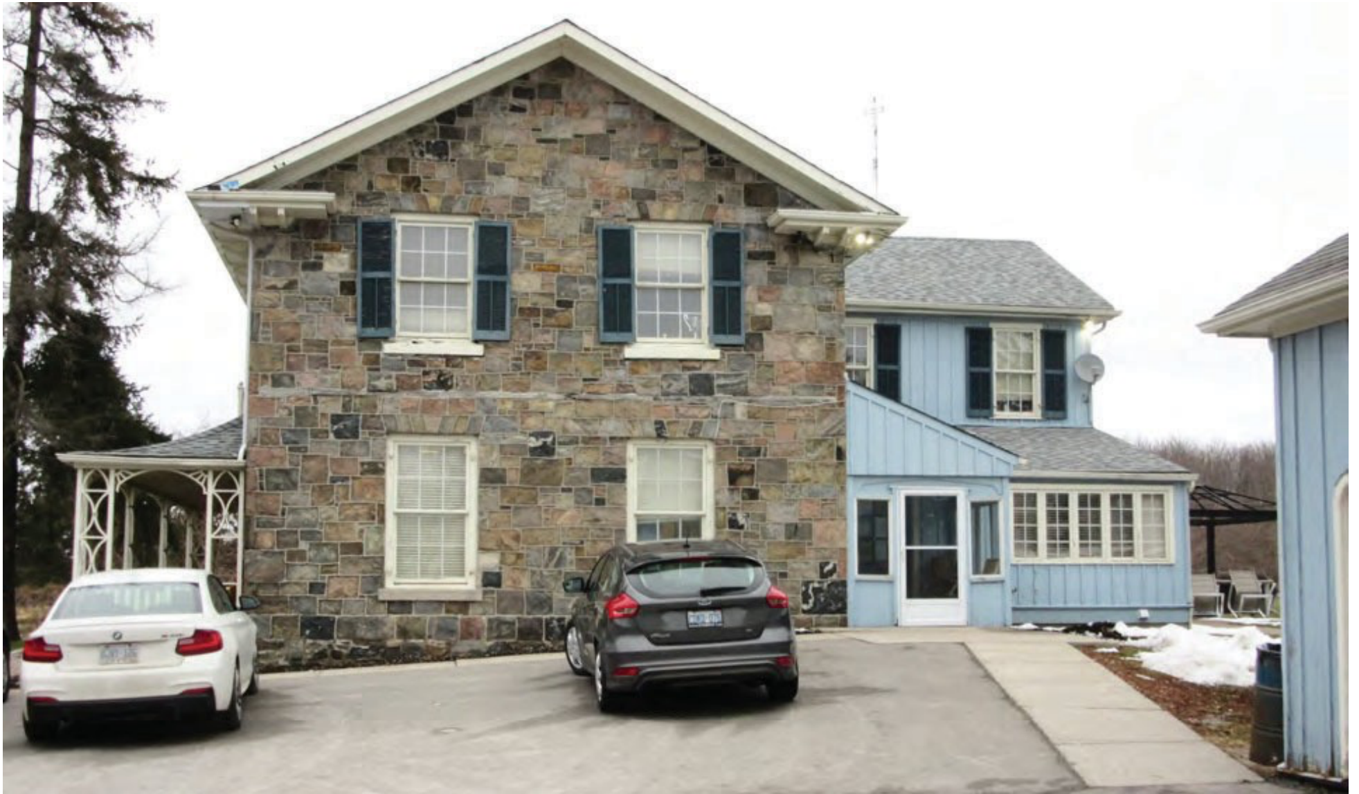
VIEW OF SOUTH ELEVATION
