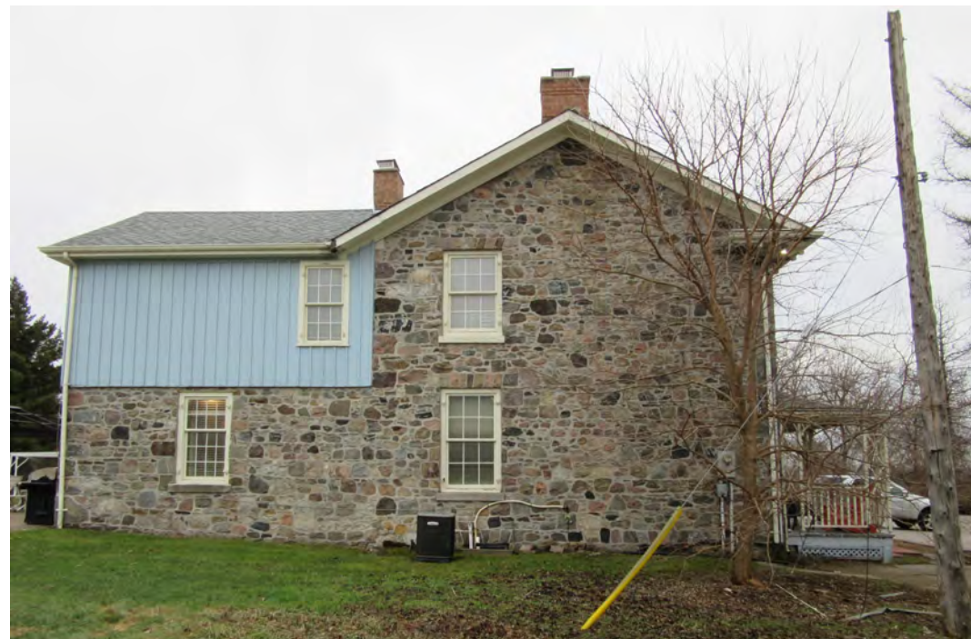
Figure 5:: view of side/north face.
