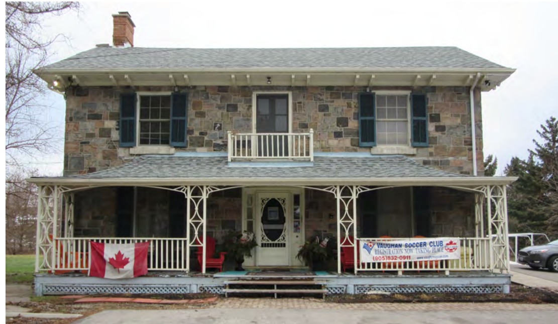
Figure 4:: view of front/west (street) face.
