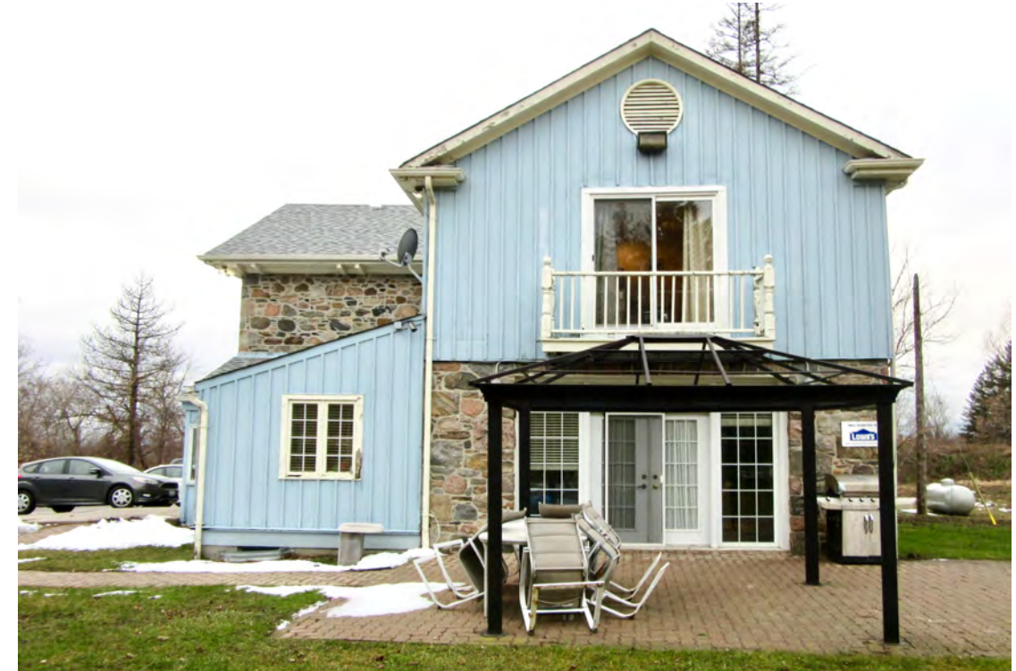
Figure 6:: view of rear/east face
