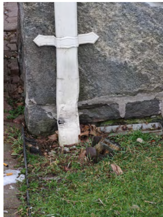
Figure 10: damaged aluminum RWL, too close to masonry. Figure 11: temporary animal infiltration screen
