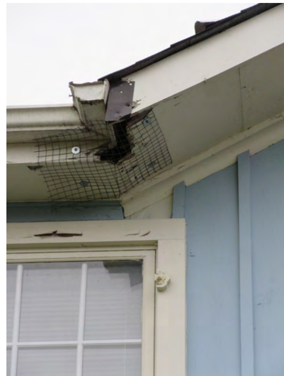
Figure 10: damaged aluminum RWL, too close to masonry. Figure 11: temporary animal infiltration screen
