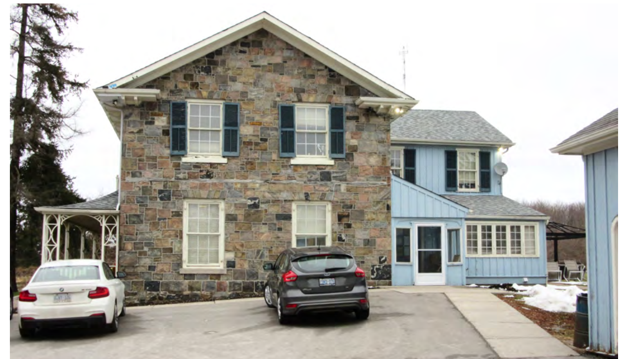
Figure 7: view of side/south face with squared stone, raised pointing, wood nailer for removed wrap-around porch.
