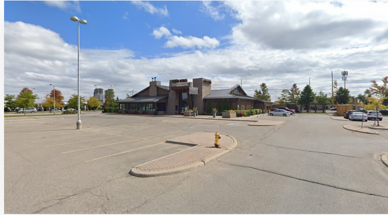
Southeast View of Subject Site - the Keg Steakhouse + Bar
