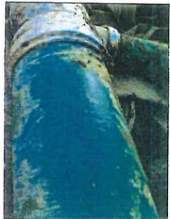
SANITARY LEAKAGE @ TEE CONNECTION
