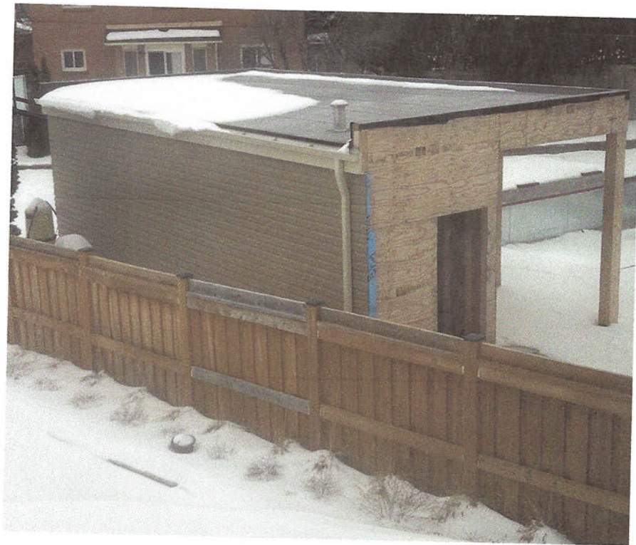
Full view of cabana from upstairs windows
