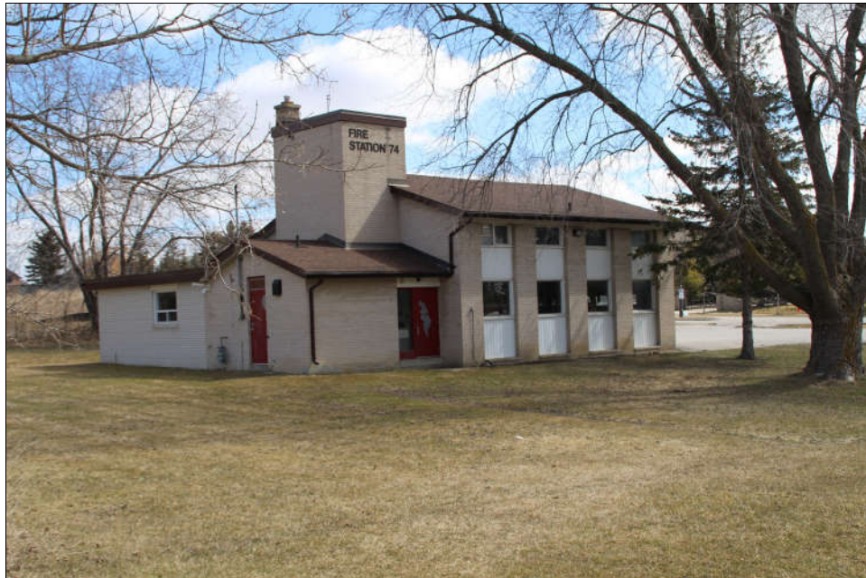
Figure 5 fire station, east side of Islington Avenue
