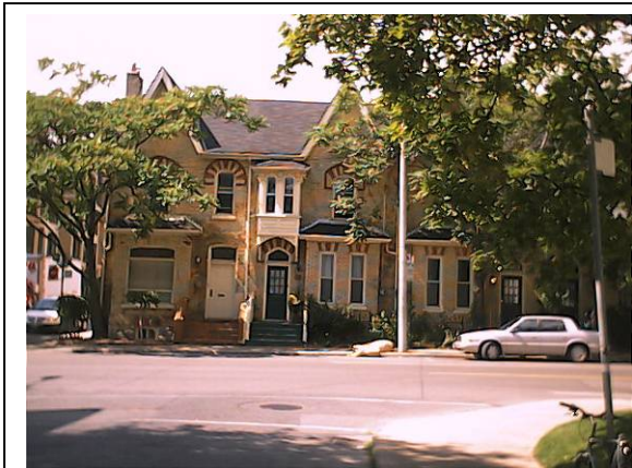
The Beverley Street project preserved a large Victorian row of 16 houses, maintaining their original use as single-family dwellings. It was nominated for an Ontario Renews Award.
