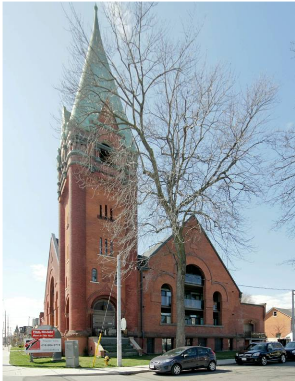
Balconies behind the original arches double the window area to meet the requirements of residential use, without cutting new openings in the historic masonry structure.
