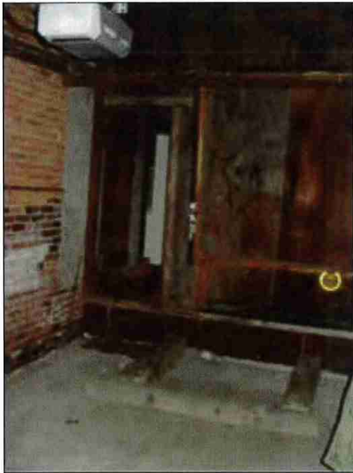
Photograph No. 37 Shed facing south with tail wing wall on left.
