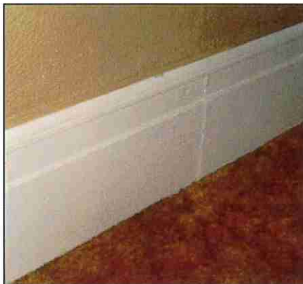
Photograph No. 19 Ground Floor South Room, detail of baseboards,
