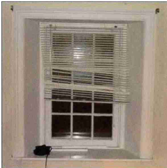
Photograph No. 31 2 nd Floor – typical window.
