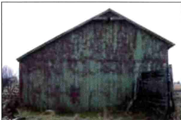
Photograph No. 4 Outbuildings – north elevation.
