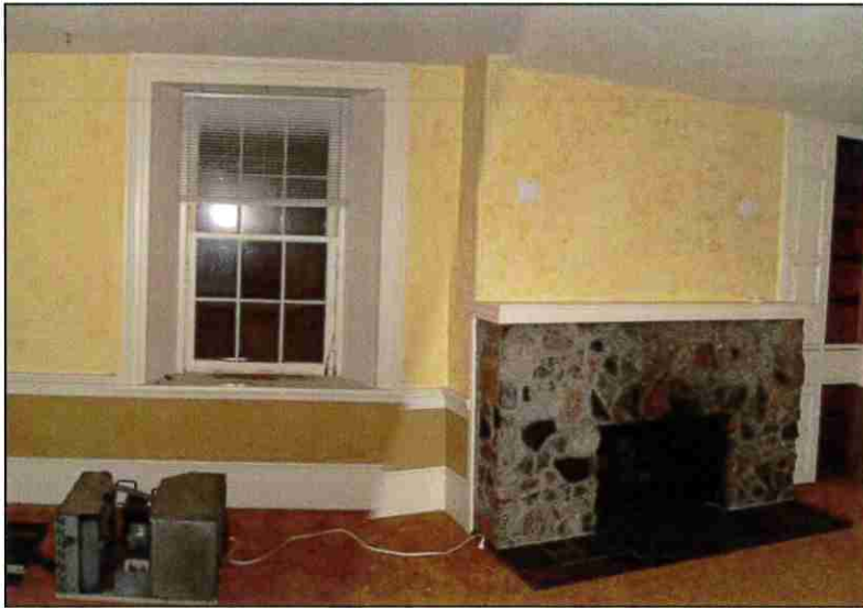
Photograph No. 20 Ground Floor, South Room – South Wall.
