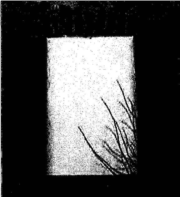
Photograph No. 10 Typical Window Opening, Side Elevations.
