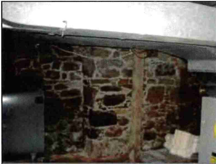
Photograph No. 24 Basement – South Room chimney pier on south wall.
