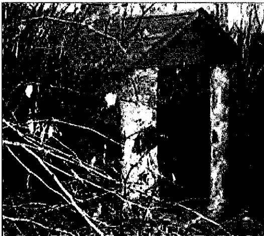
Photograph No. 12 Basement Entrance Vestibule South Elevation.
