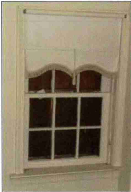
Photograph No. 34 Tail wing – 2 nd floor north elevation – window.
