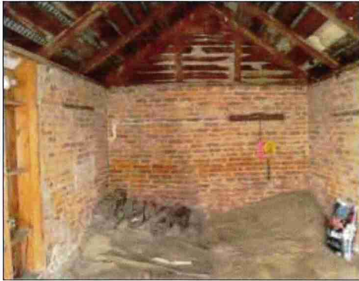
Photograph No. 5 Outbuildings – smaller structure – interior.
