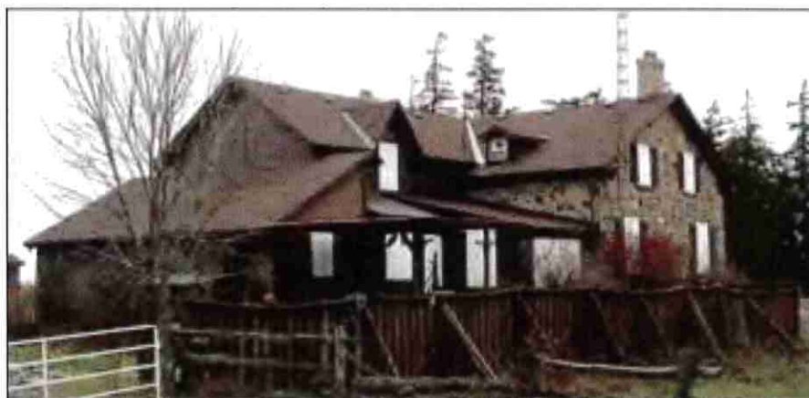
Photograph No. 5 South & West Elevations
