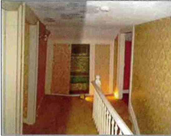
Photograph No. 26 2 nd Floor Hall looking east.
