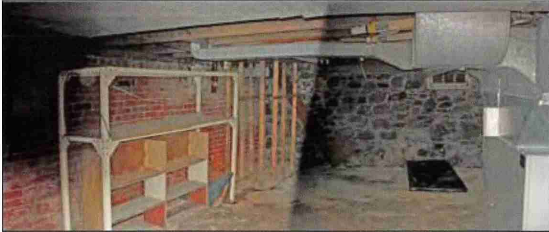
Photograph No. 23 Basement – South Room looking east
