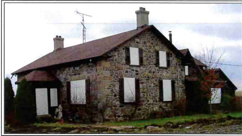
John Lawrie Farmhouse – 2005 –East and North Elevations [Source: City of Vaughan, Recreation and Culture Department].
