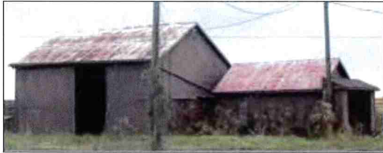
Photograph No. 1 Outbuildings – west and south elevations
