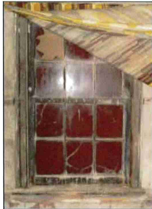
Photograph No. 33 Tail wing – ground floor south elevation – original window.
