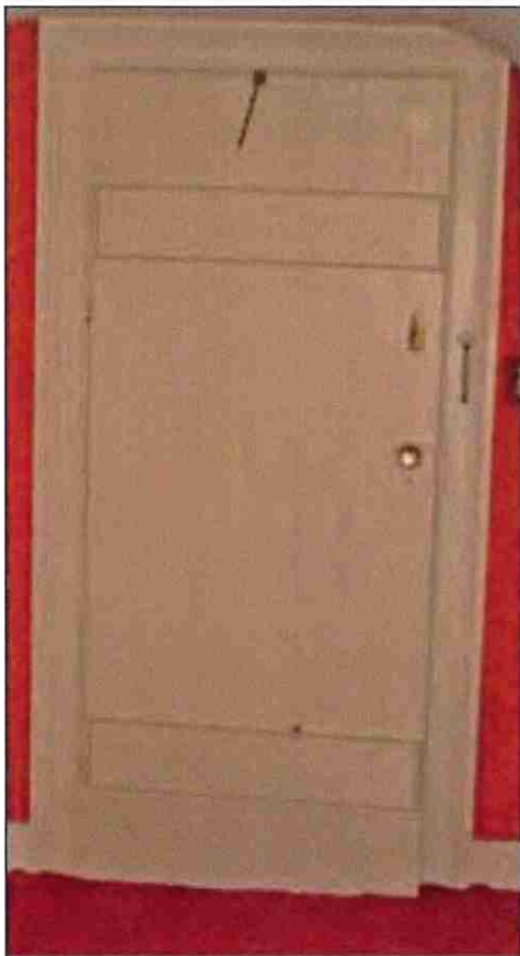
Photograph No. 28 2 nd Floor – typical board door.
