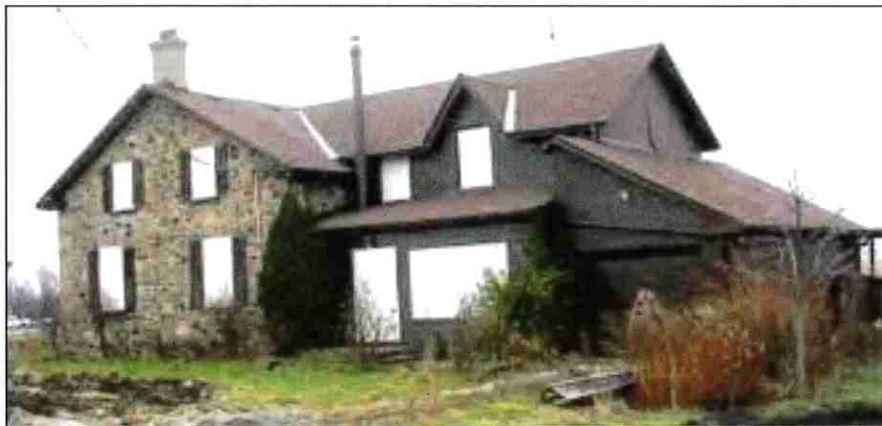
Photograph No. 4 North & West Elevations.
