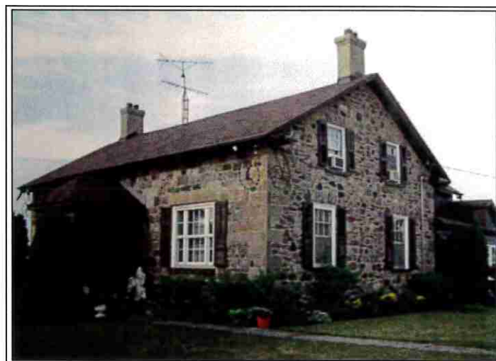
Figure 4.2 John Lawrie Farmhouse – 2005 – East and North Elevations [Source: City of Vaughan, Recreation and Culture Department].
