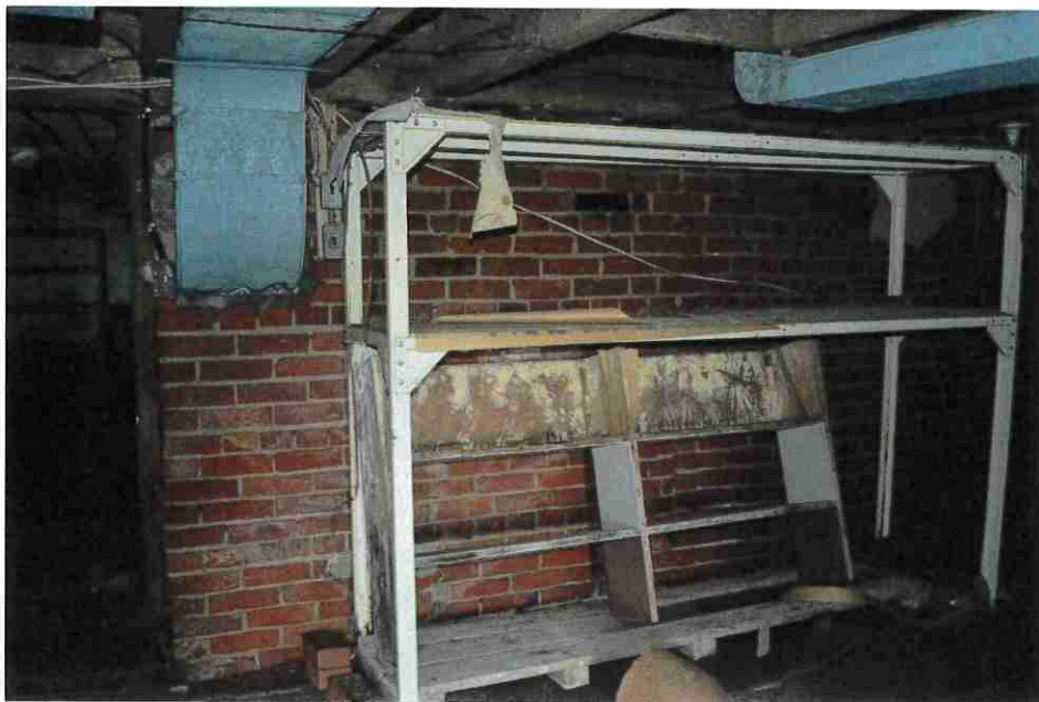
Figure 44: Brick wall under summer beam note attached to stone walls.
