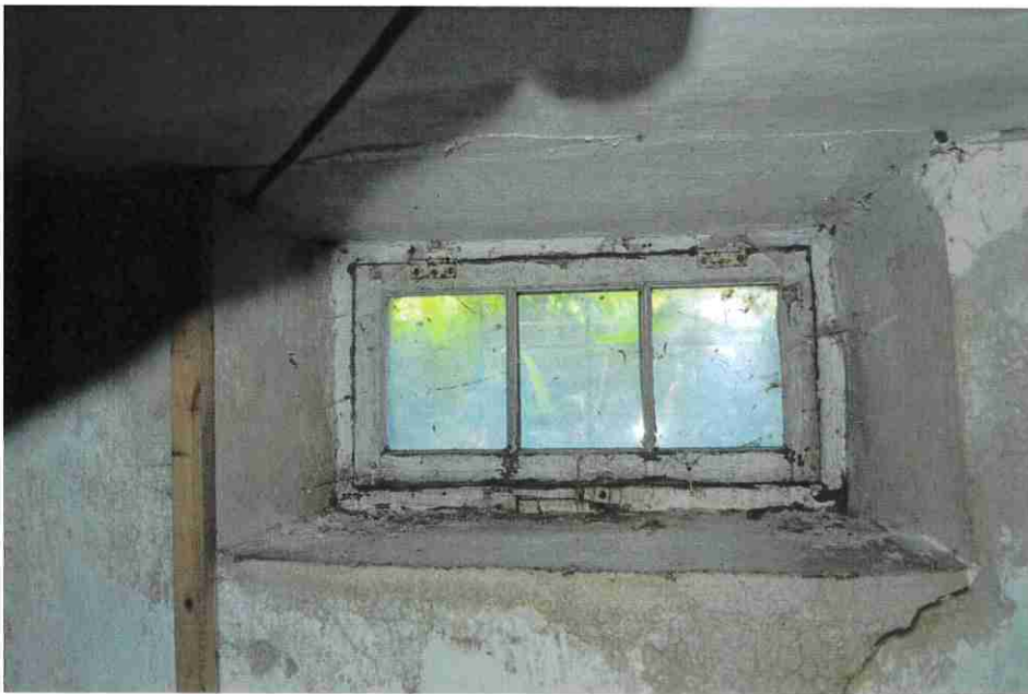
Figure 42: Cellar window North room Note Rough cast parged walls.
