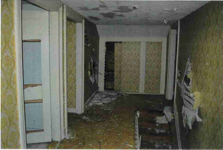
Figure 31: Second floor Hall looking west.
