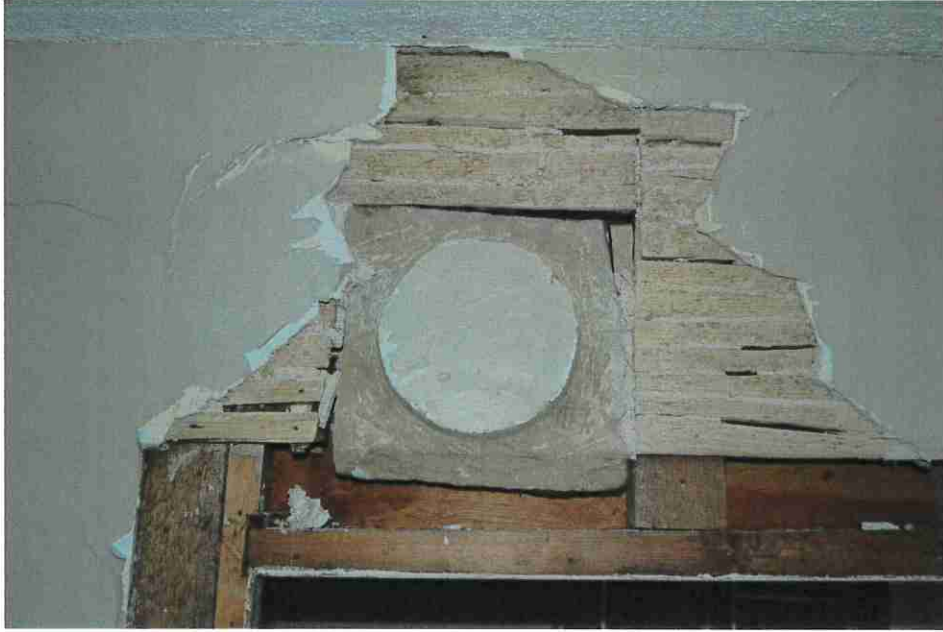
Figure 37: Stone pipe thimble support to parlour from north kitchen.
