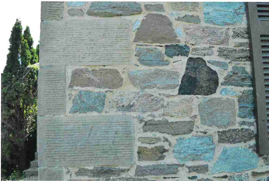
Figure 48: Stonework on north wall random rubble granite.
