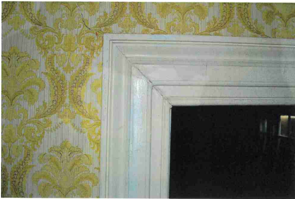
Figure 34: Ground floor door casing.
