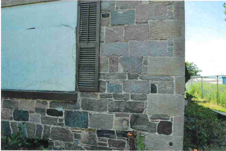
Figure 47: Coursed granite stone work with tooled limestone quoins.
