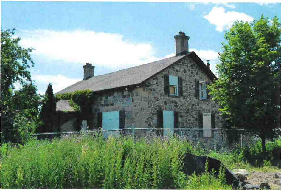
Figure 11: View to south west from drive.
