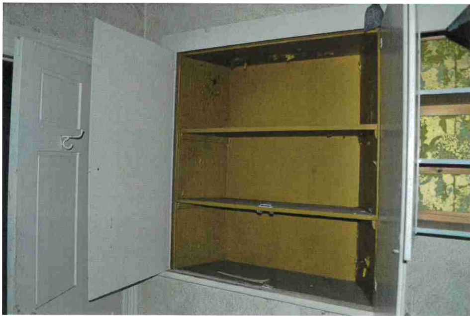
Figure 36: North west kitchen - Window in wall used as a cupboard.
