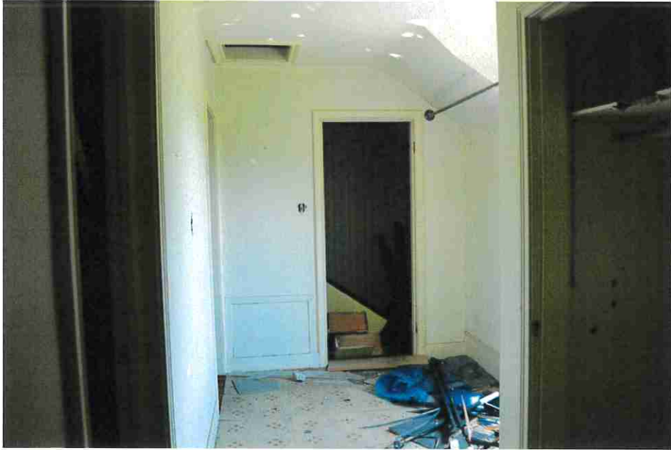
Figure 51: Brick addition hall looking east.
