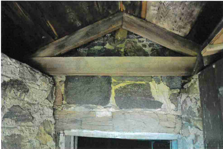
Figure 38: Roofing framing to cellar entrance.
