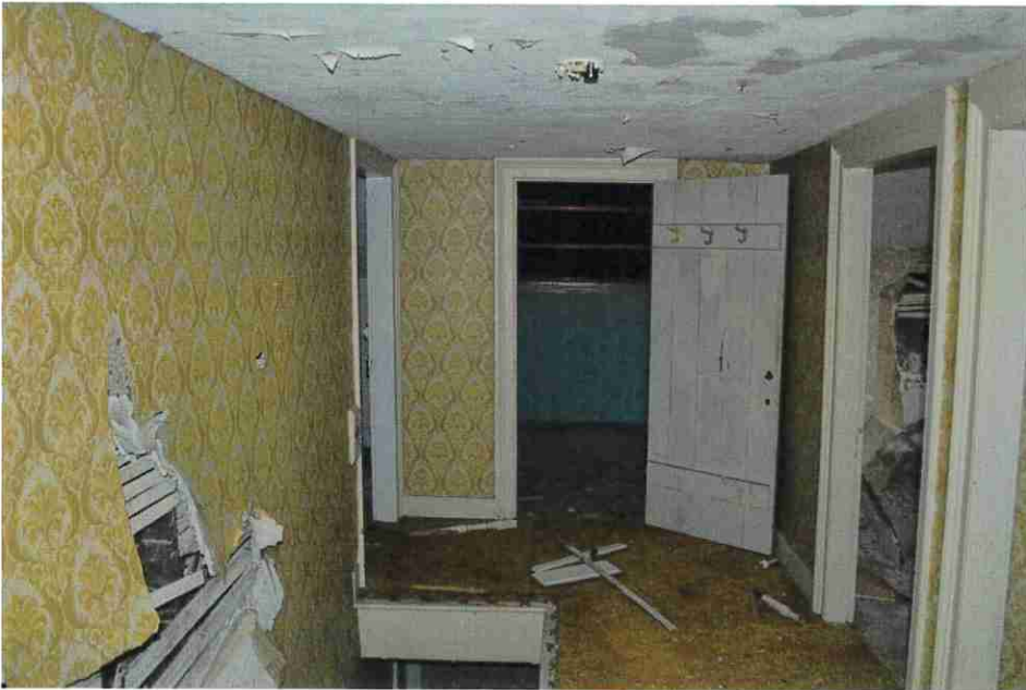
Figure 32: Second floor Hall looking east.
