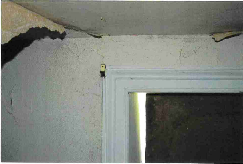
Figure 33: Detail of second floor window casing.
