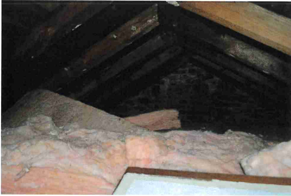
Figure 45: Attic framing. Note offset chimney.
