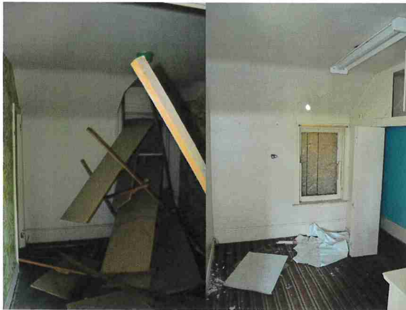
Figure 52: Brick addition second floor west and east bedrooms.
