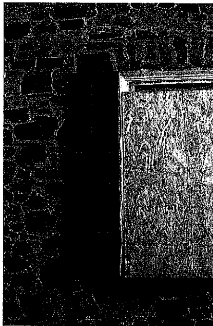
Figure 54: Original shutter screwed to wall. Note: Shutter is upside down and on the wrong side
