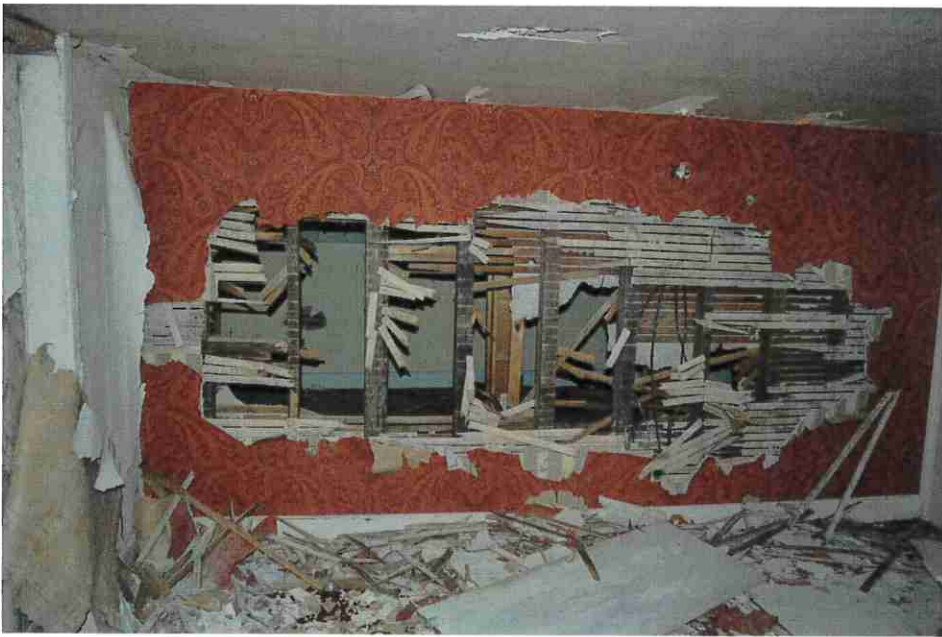
Figure 28: Stud and lath of north bedrooms.
