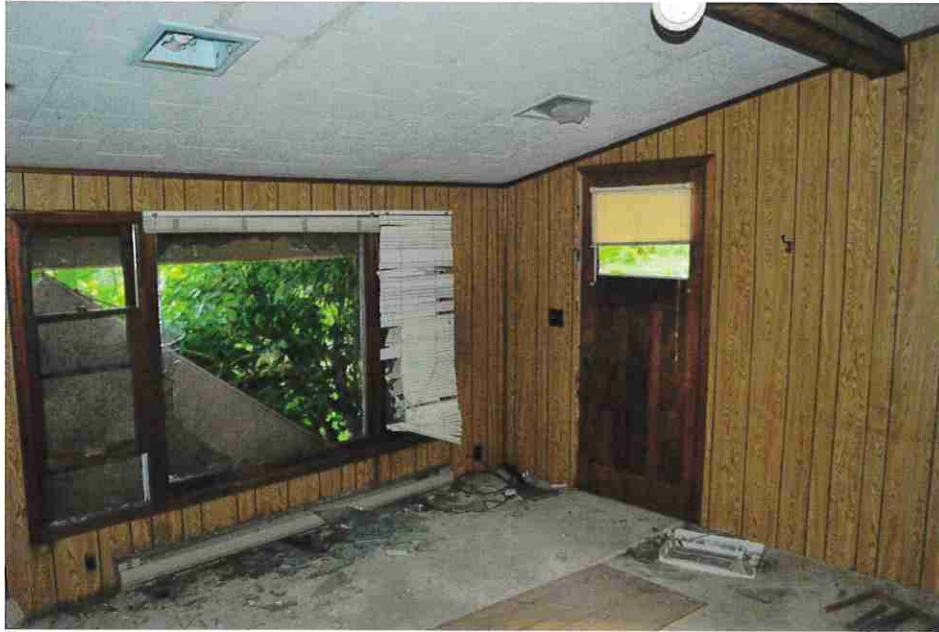
Figure 49: Enclosed south porch.
