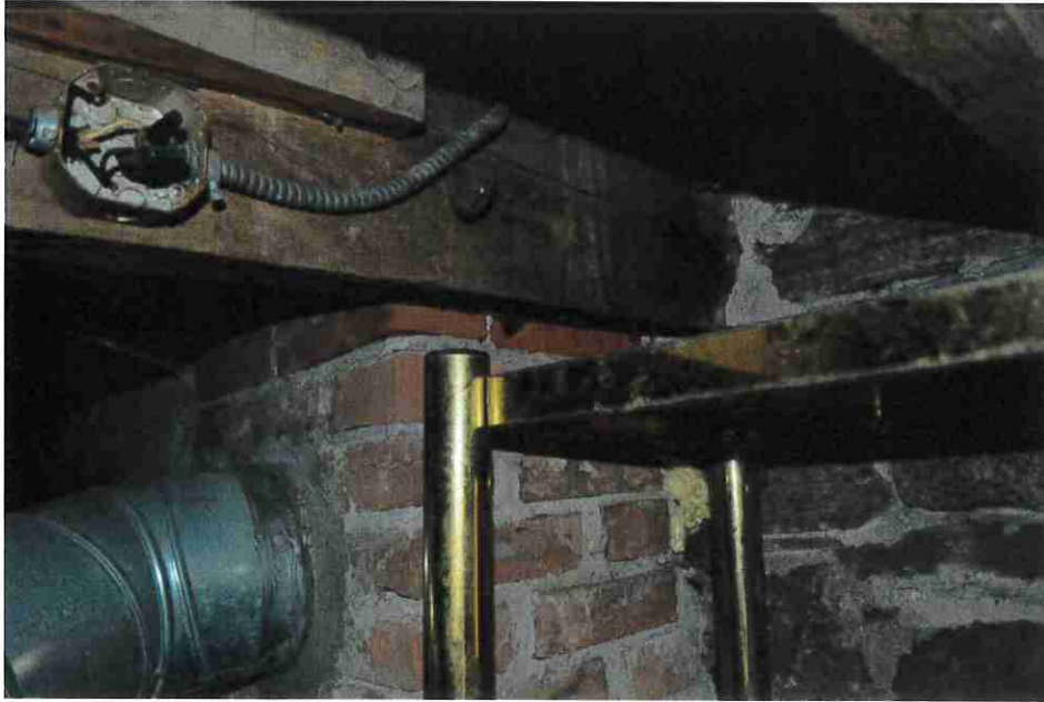
Figure 41: 3" by 10" Floor Joists at 24" set into stone south side.
