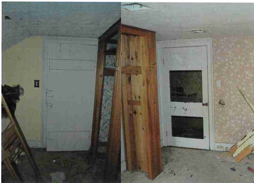
Figure 30: North and south bedroom doors. Note plank north doors compared to six panel south bedroom doors.
