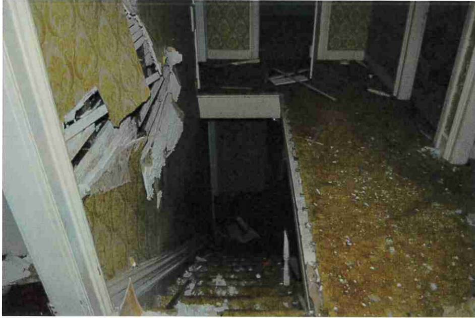
Figure 25: Stair from second floor hall.
