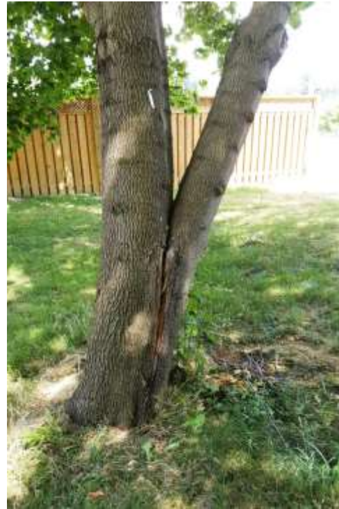
Tree #091. Located just north of gravel driveway. Tree is splitting apart and is in a hazardous condition.
