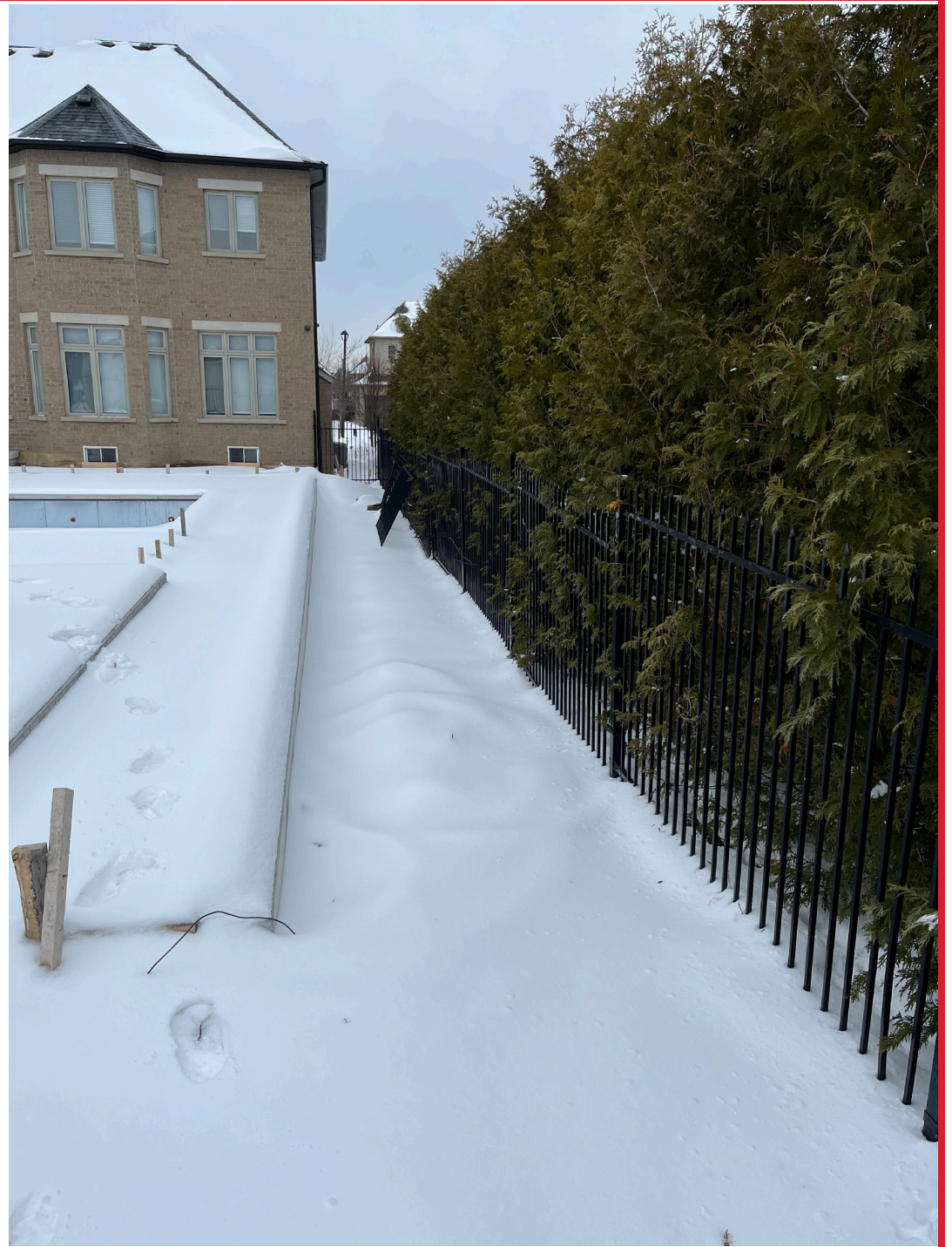
View along south lot line - showing existing retaining wall
