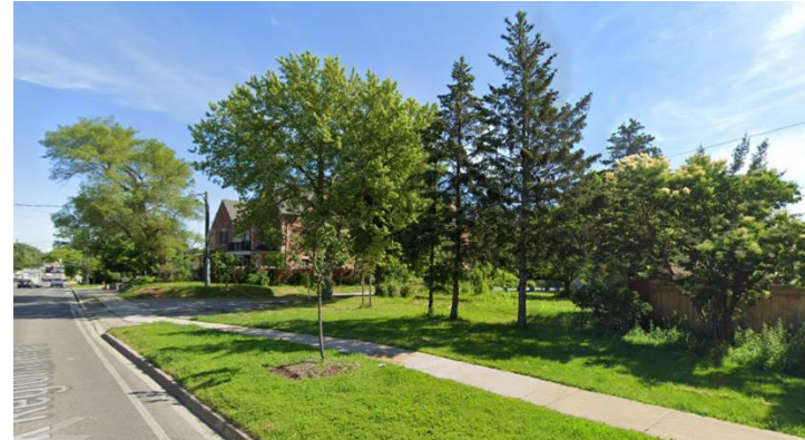
Figure 9 - View of front of subject property from southwest (Photo: RHC 2020)
