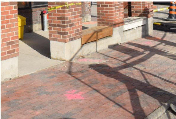
Photo 7: Brick and concrete walkway and benches between colonnade, looking east
