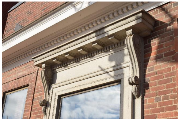
Photo 12: Cornice and door surround details, looking north
