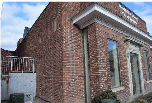
Photo 25: West façade, looking northeast
