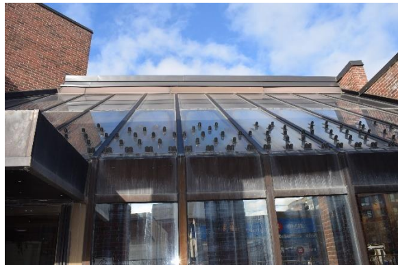
Photo 18: Skylight, looking north
