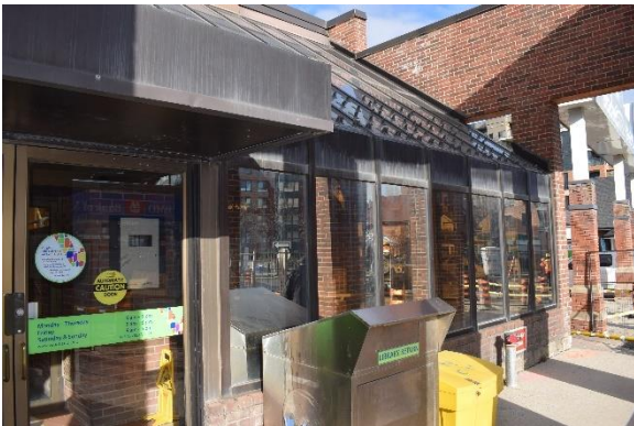
Photo 17: Skylight and windows, looking east
