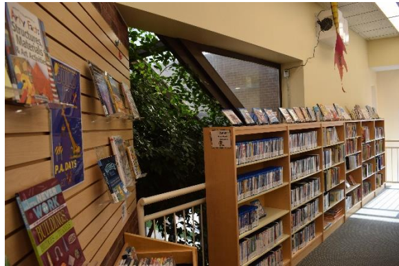
Photo 38: Fixed window looking at colonnade, looking south
