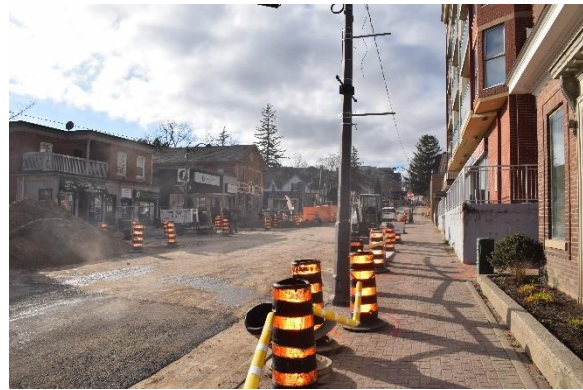
Photo 2: Woodbridge Avenue, looking west
