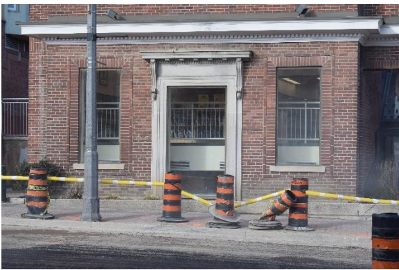
Photo 13: Window openings and door surround, looking north
