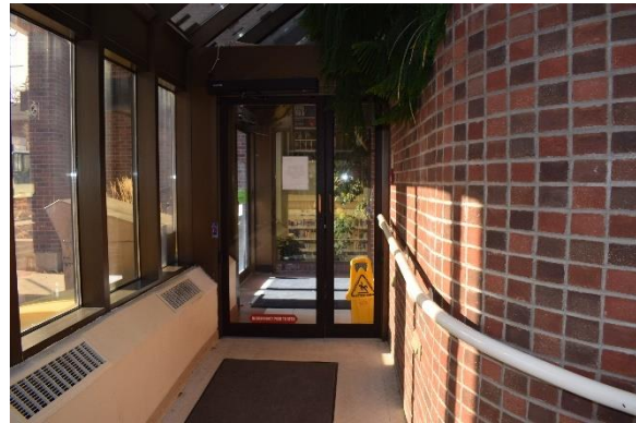
Photo 28: Door between main entrance and ramp, looking west
