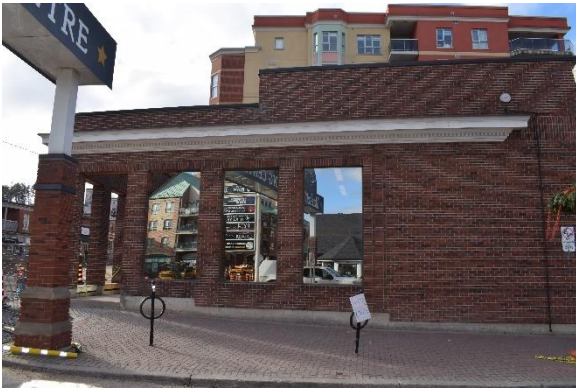
Photo 21: East façade east part, looking west at cornice and windows
