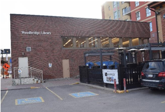
Photo 23: North façade, looking south
