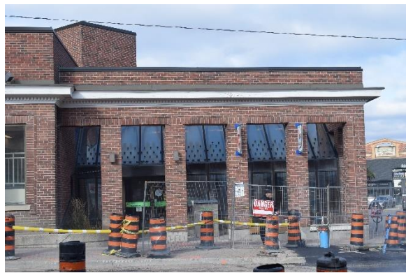
Photo 14: East section of front façade, looking north
