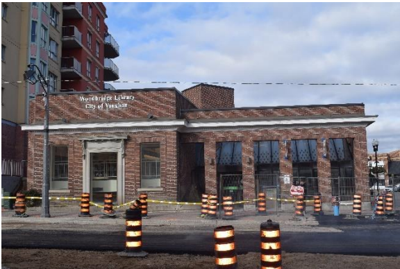
Photo 9: Front façade of structure, looking north
