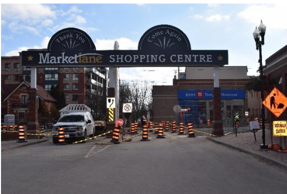
Photo 3: Access Road to Market Lane Centre, looking south
