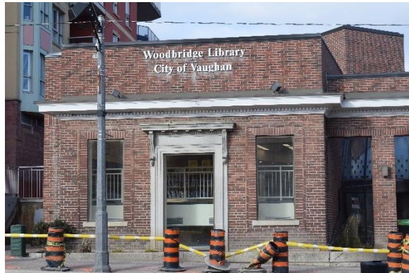
Photo 10: Front façade of west section, looking north
