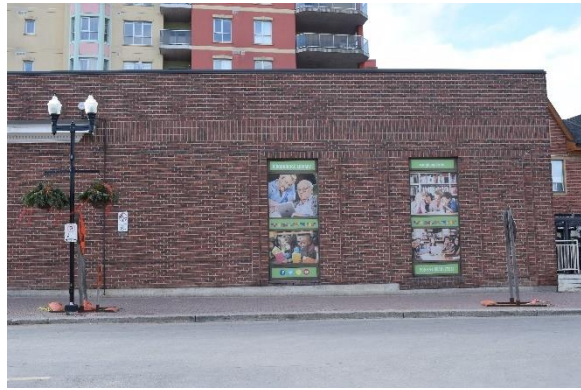
Photo 22: East façade, looking west at window openings and belt course
