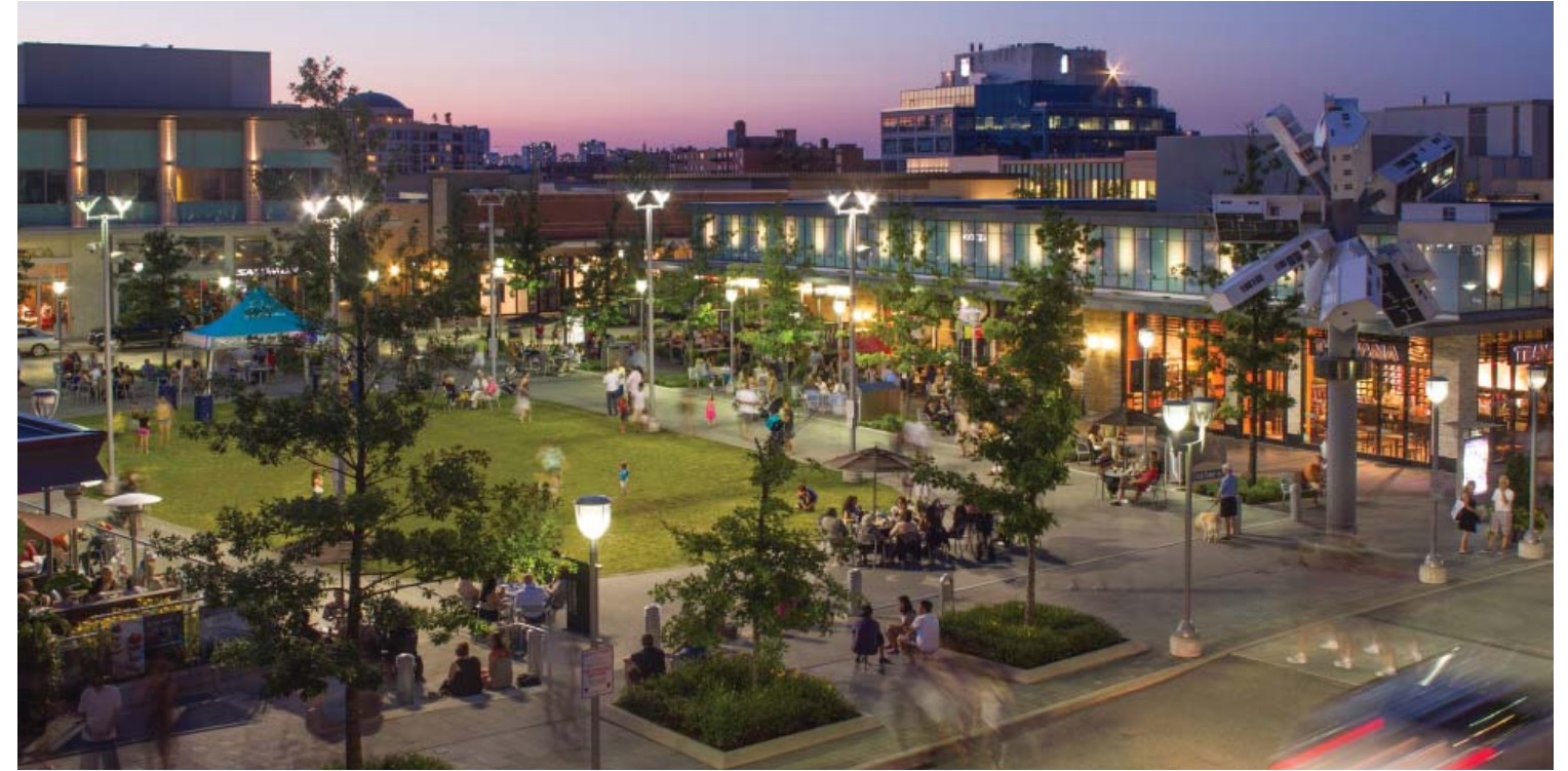
SHOPS AT DON MILLS, TORONTO
