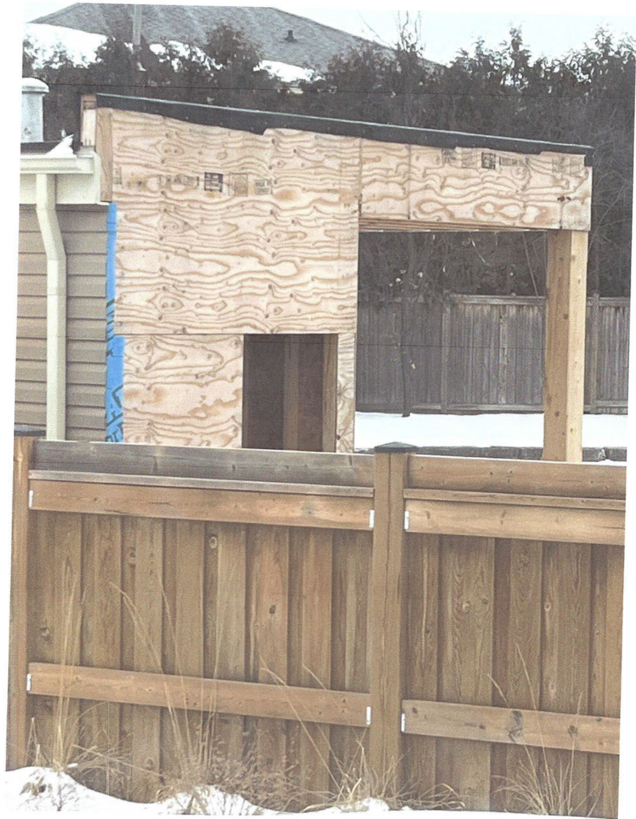
View of cabana washroom doorway from kitchen windows
