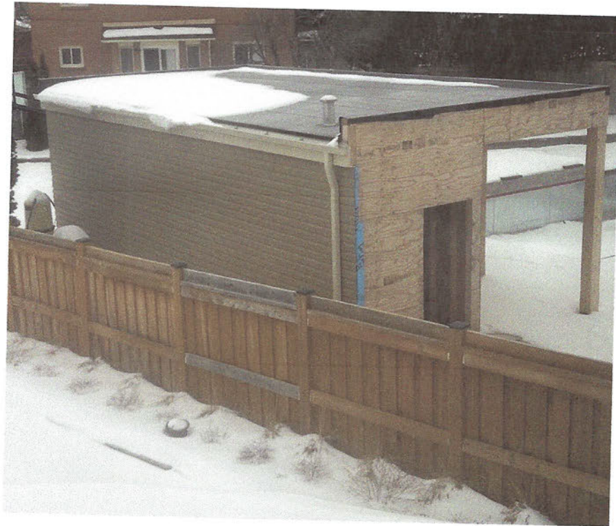
Full view of cabana from upstairs windows
