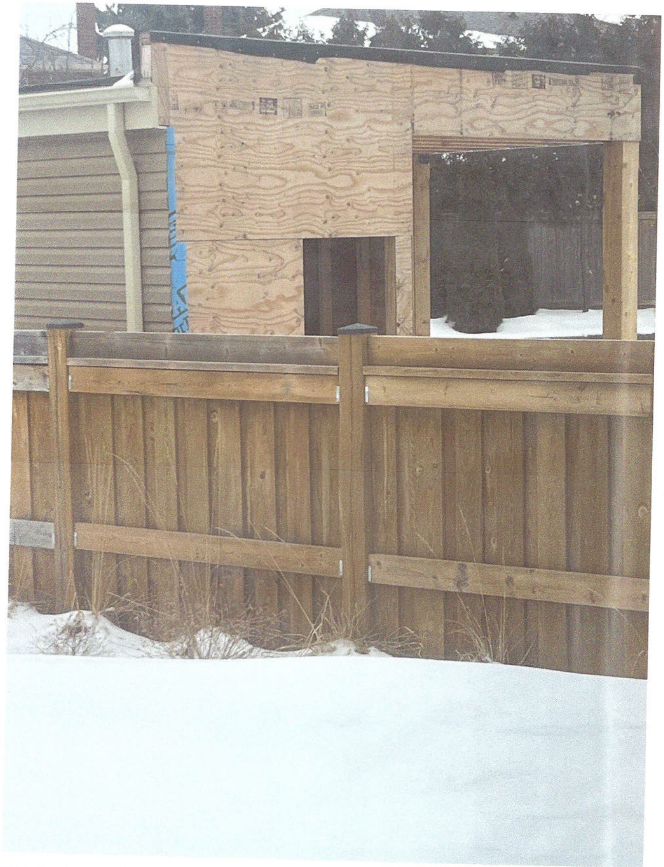
View of cabana washroom doorway from family room windows
