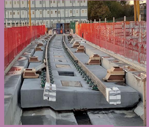
Examples of Floating Slab Track
