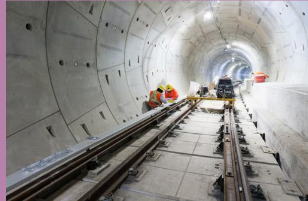
Examples of Floating Slab Track
