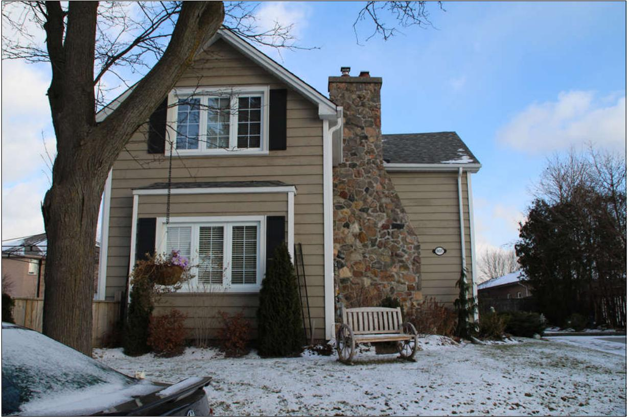
Figure 7 9697 Keele - front (west) elevation - front wing & fieldstone chimney are later additions
