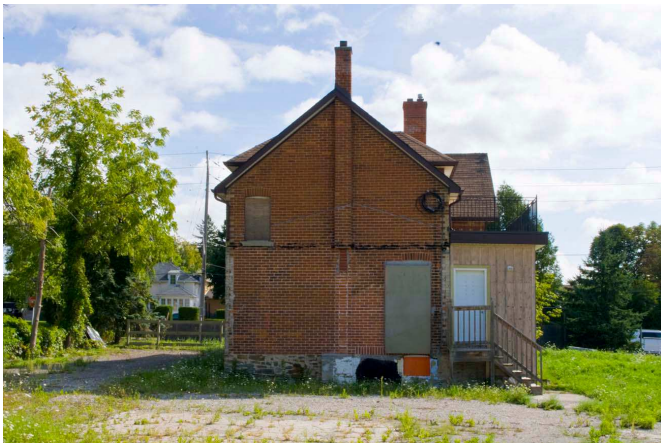
Photo 3 Looking To West Side
