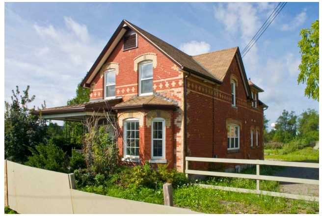
Photo 2 Looking To North-East Corner
