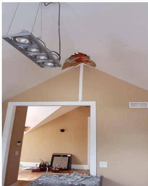
Photo 11 2x8 Rafters on 12" Ridge Beam
