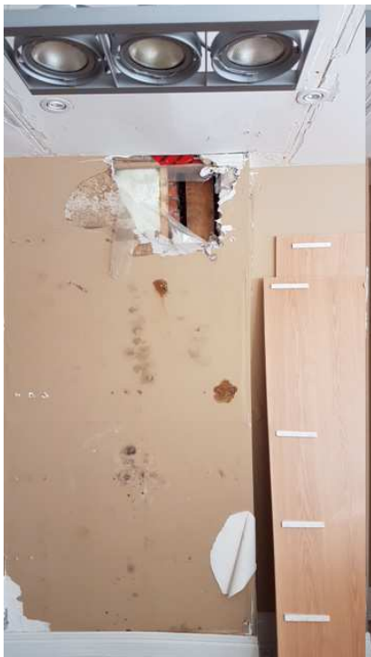
Photo 5 - 2x8 Joists 2 nd Floor - Living/Dining/Reception
