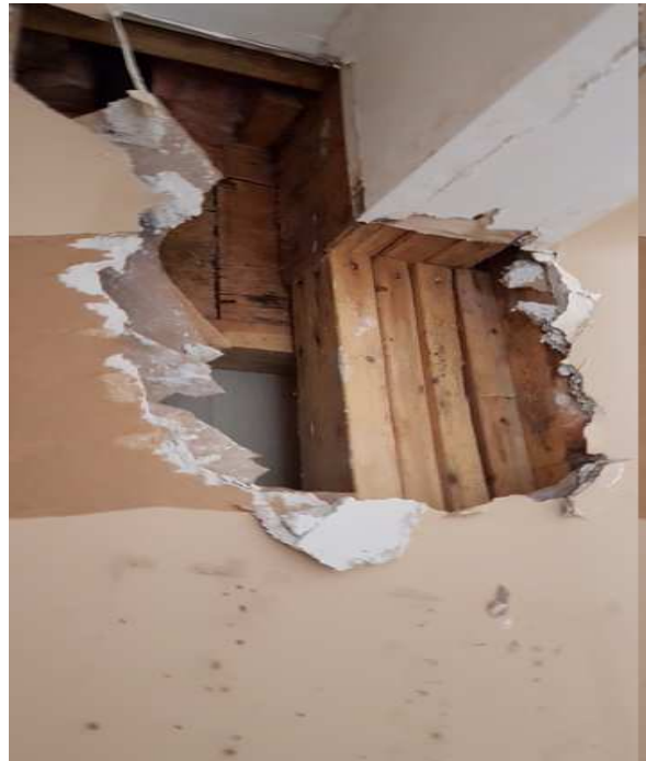
Photo 8 - 4 ply 2x10 Beam Main Floor Powder Room
