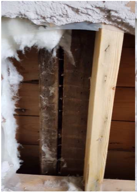
Photo 5 - 2x8 Joists 2 nd Floor - Living/Dining/Reception
