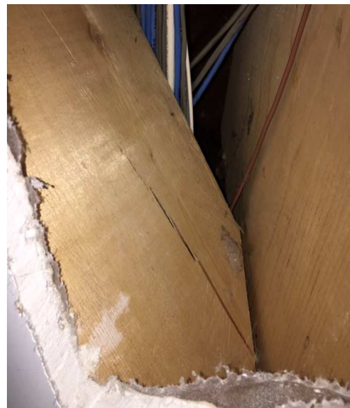
Photo 12 2x8 Rafters on 12" Valley Beam
