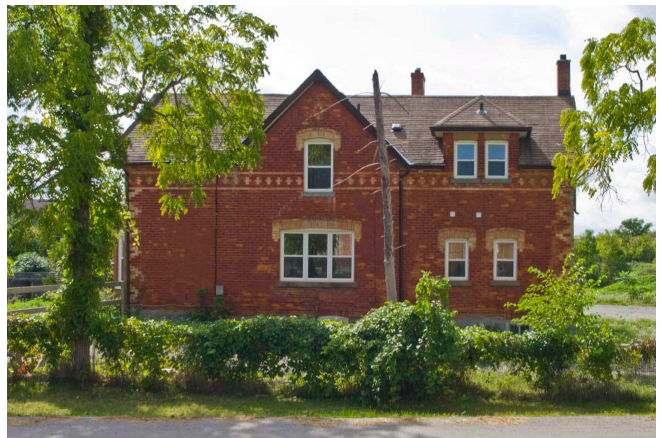
Photo 4 Looking To West Side
