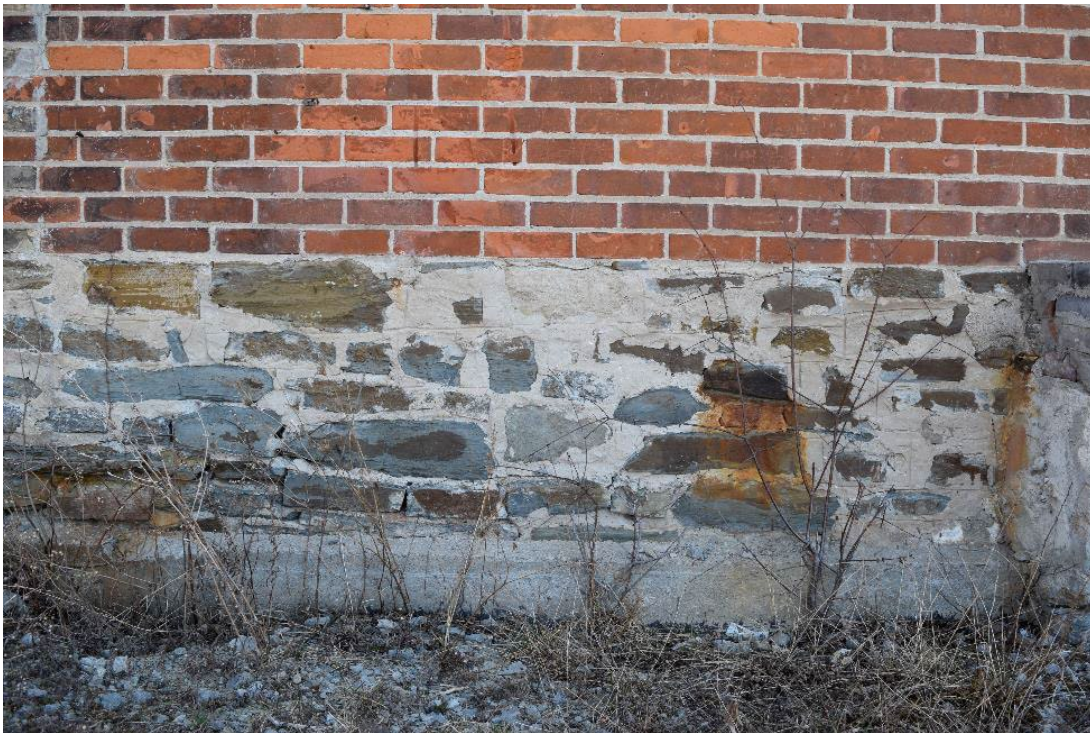
Image 20: Example of field stone foundation with flush bond mortar
