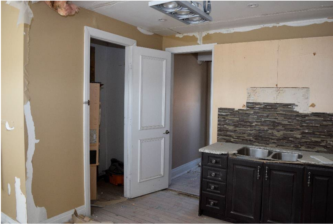
Image 35: Kitchen on first floor, facing southwest
