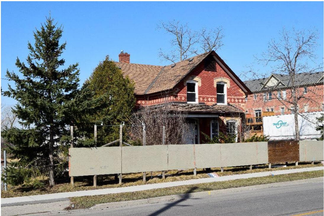
Image 7: Southeast corner of Moody-Darker House, facing northwest
