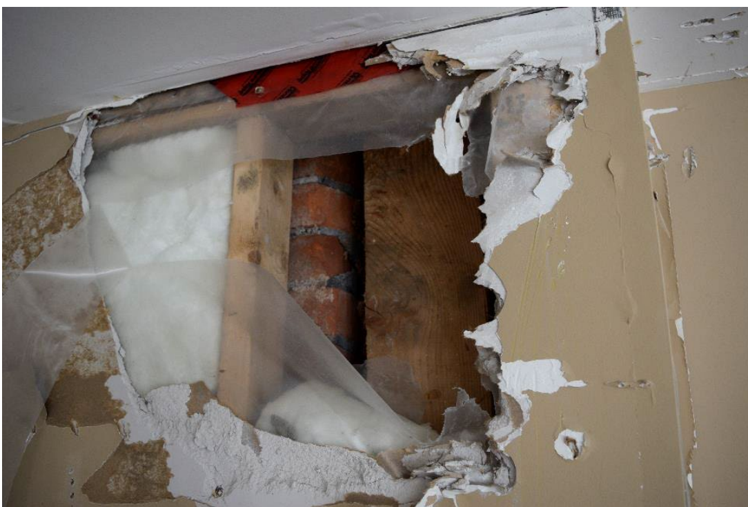
Image 44: Example of new wall framing with original brick behind
