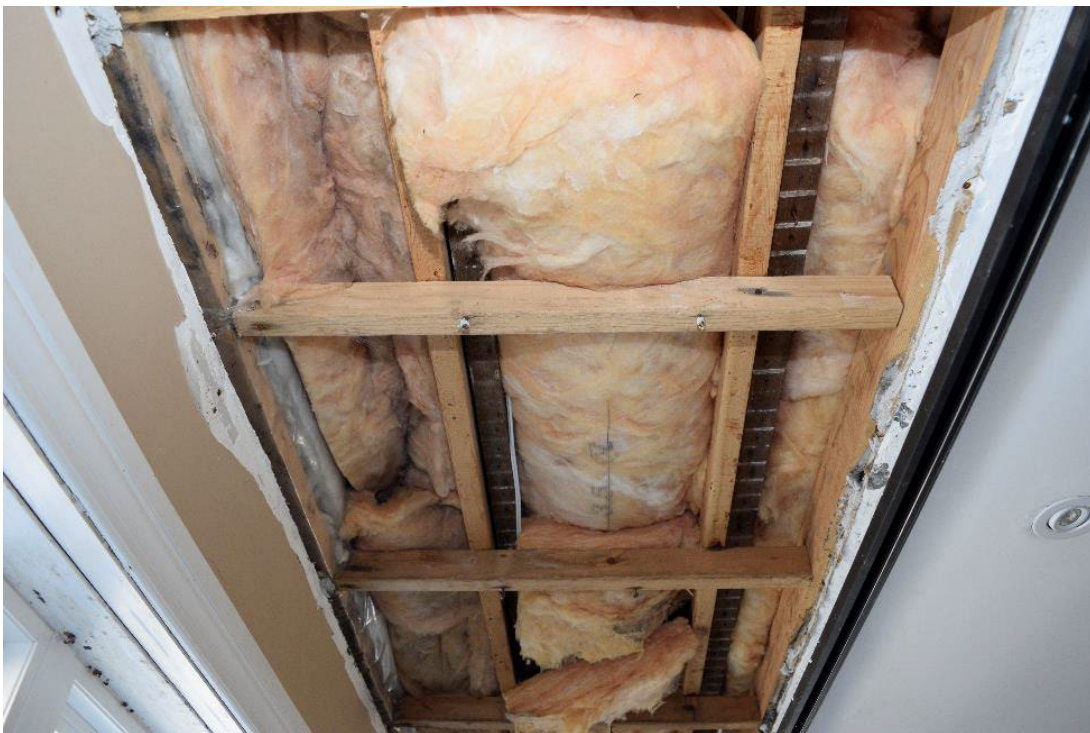
Image 33: Evidence of past renovation, note use of sistered joists
