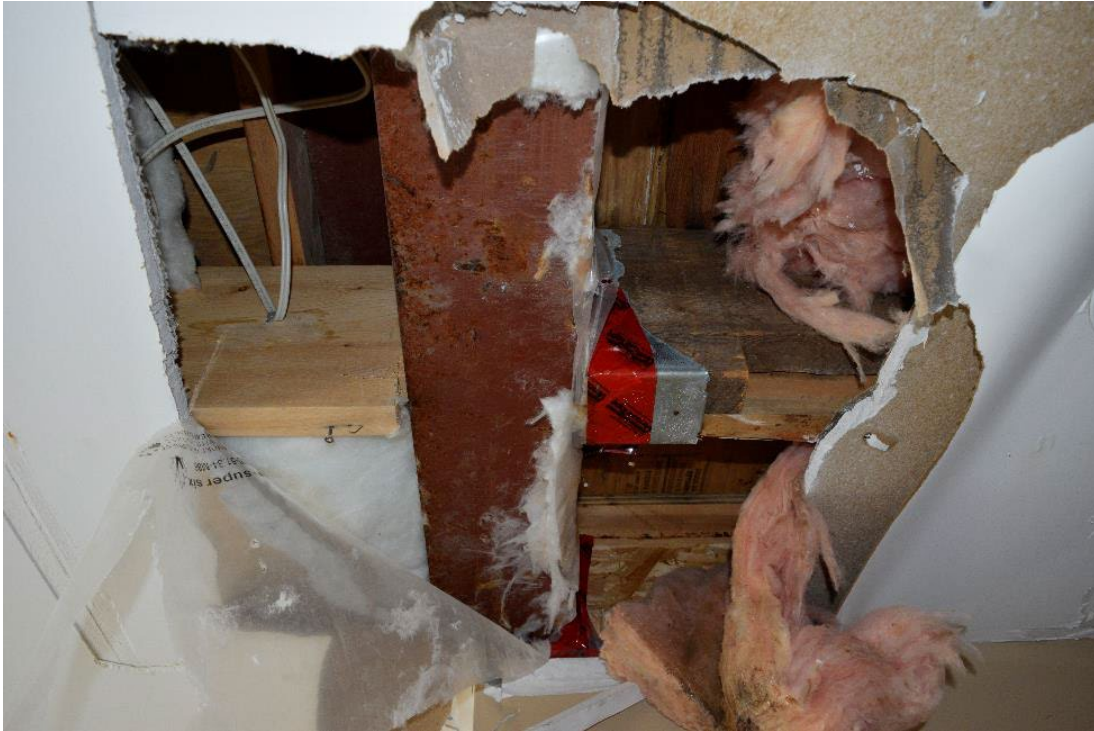
Image 37: Steel I-beam used to replace structure where wall has been removed
