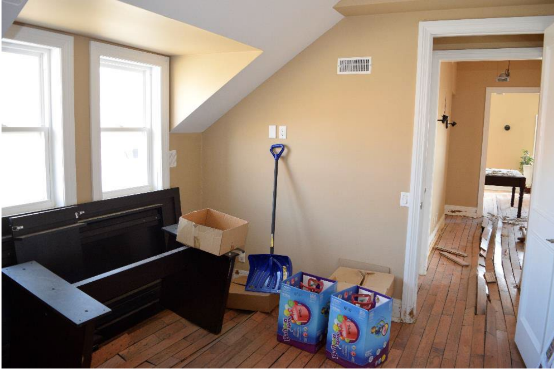
Image 41: Rear room on second floor, facing north, windows are located in hip dormer depicted in Image 25, note water damage to flooring
