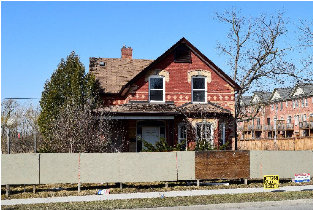
Image 1: Front façade of Moody-Darker House, facing west
