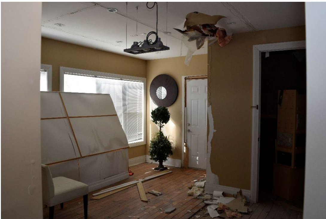
Image 36: Area where large section of wall has been removed, facing southwest
