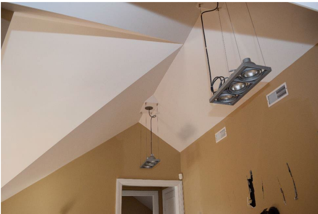
Image 40: Modern roof construction on second floor
