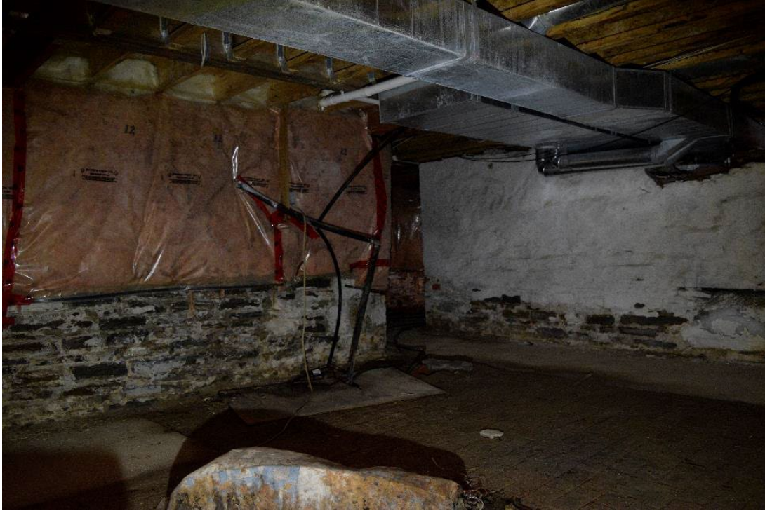
Image 49: Overview of basement
