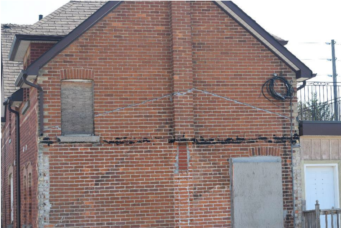
Image 21: Rear of structure showing signs of removal of previous rear addition
