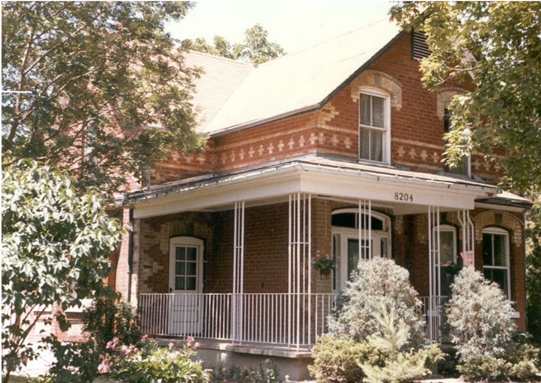
Image 51: c.1971 image of Moody-Darker House, note original windows and doors
