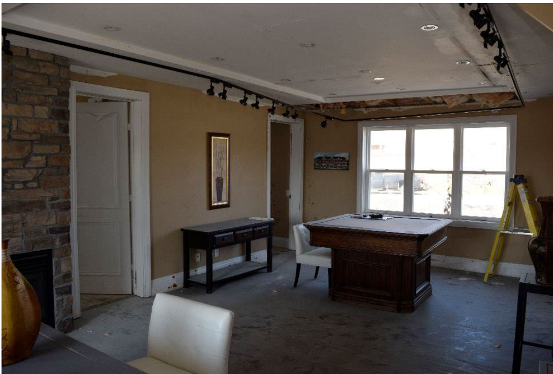
Image 31: Typical example of the interior of structure, facing north
