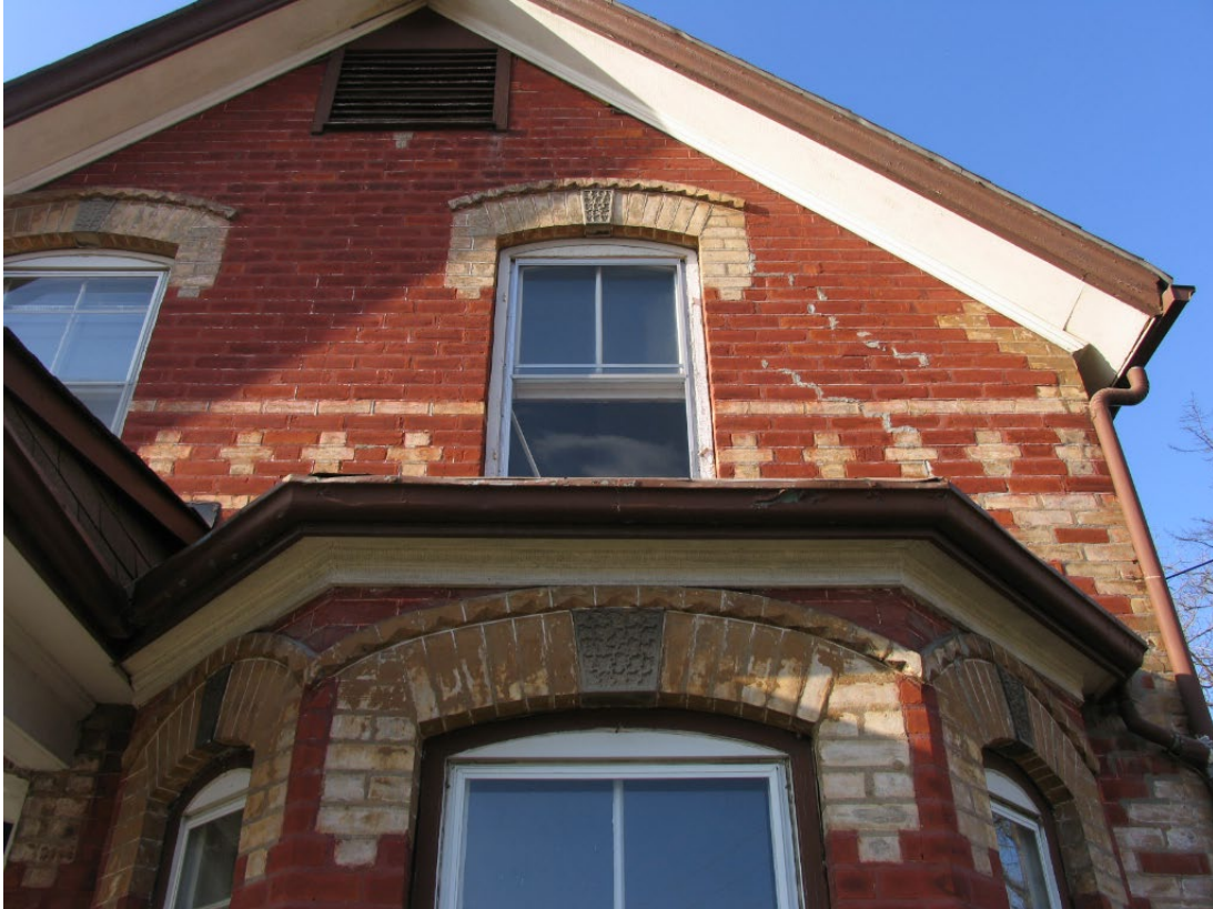
Image 53: Original moulded soffit and fascia, date of photo unknown
